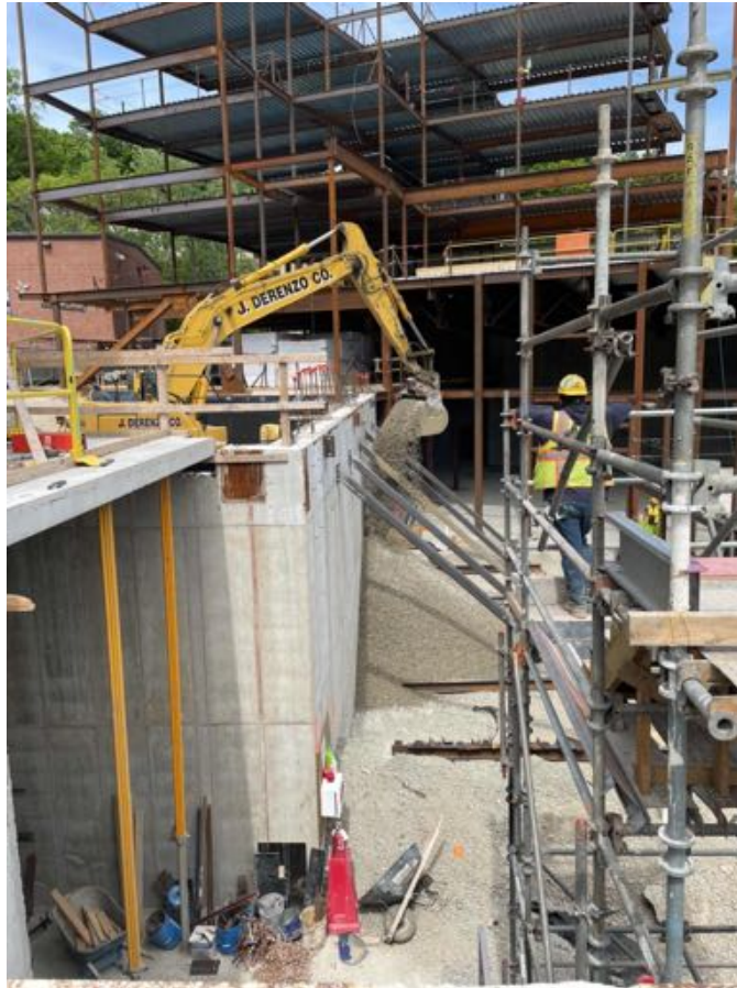
Stockpiling stone for Area A.
