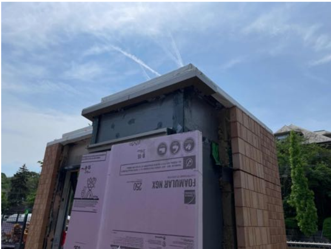
Roof edge at mock-up
