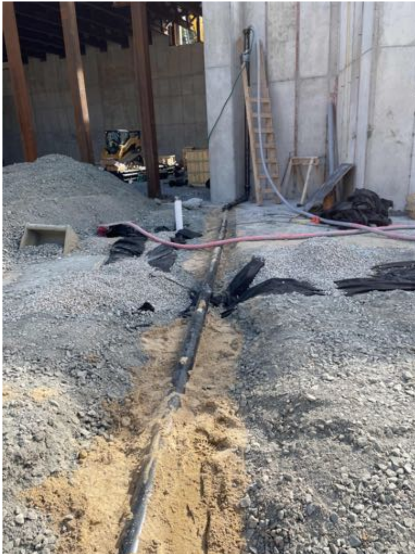
Underground plumbing inspection – passed.
