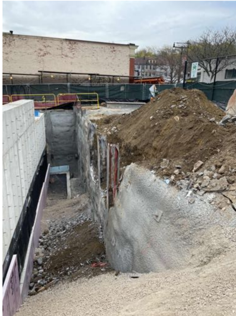
SOE demolition prior to backfill.
