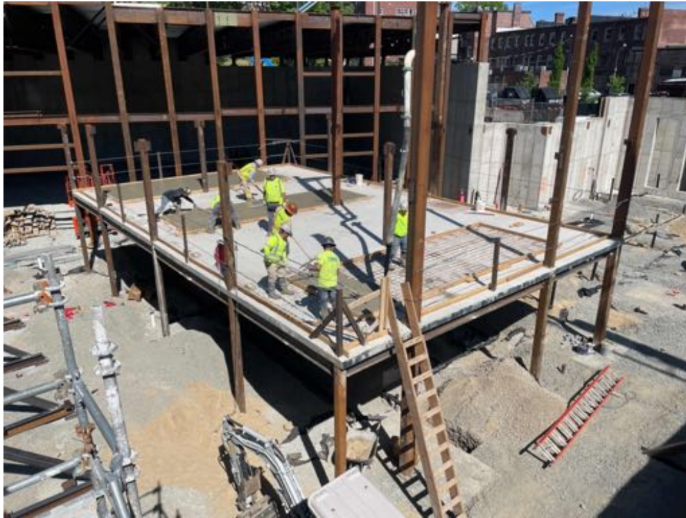
Mezz pads poured.
