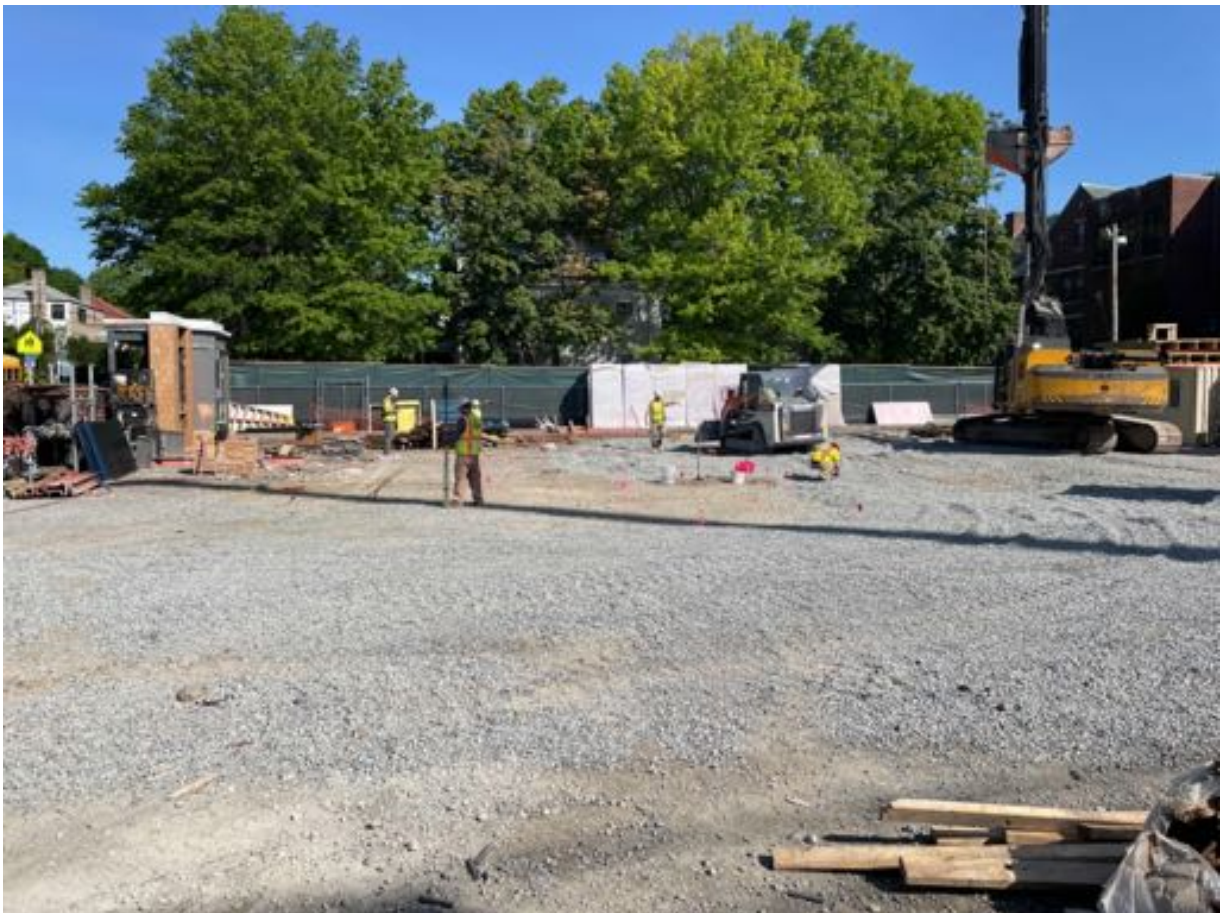
Geopier installation/layout in Area B.
