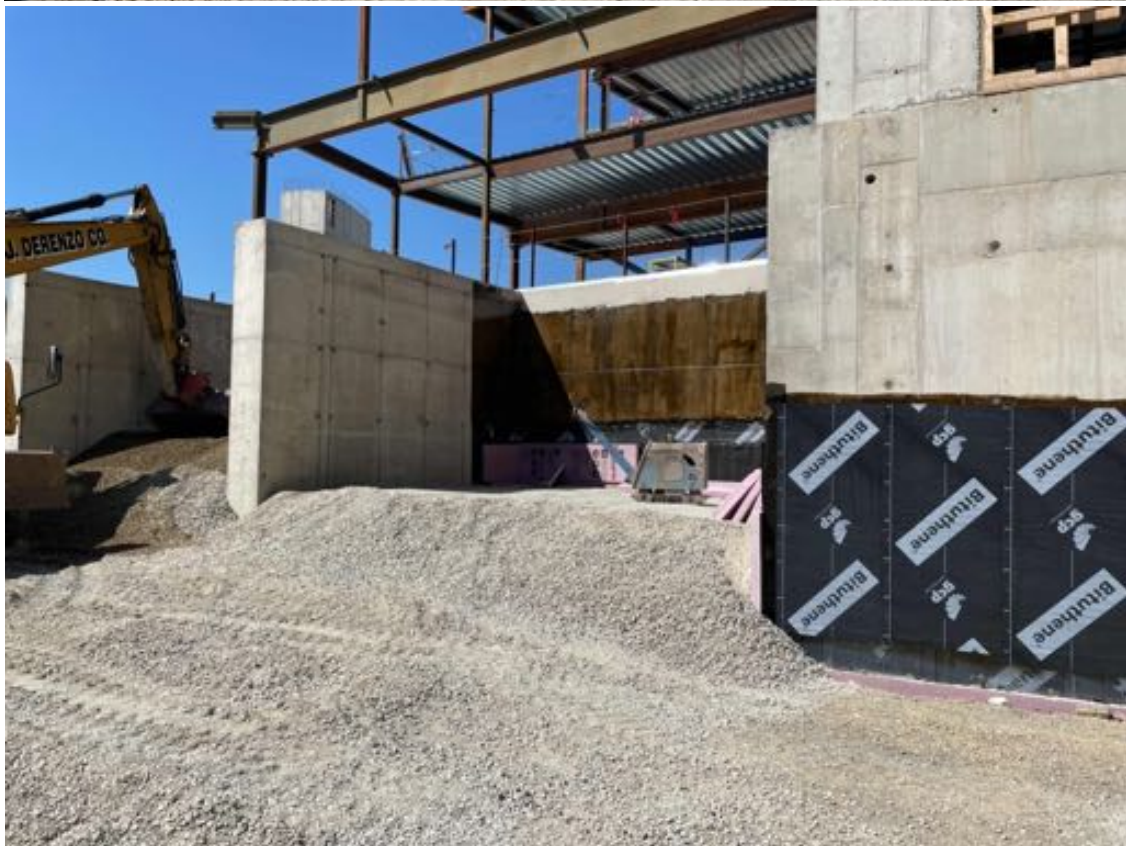
Waterproofing and backfilling, Westbourne side.
