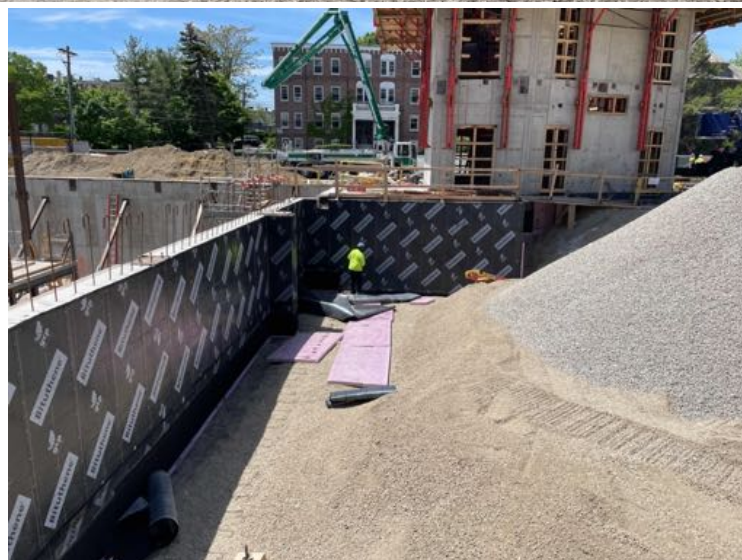
Waterproofing and backfill at line A1.
