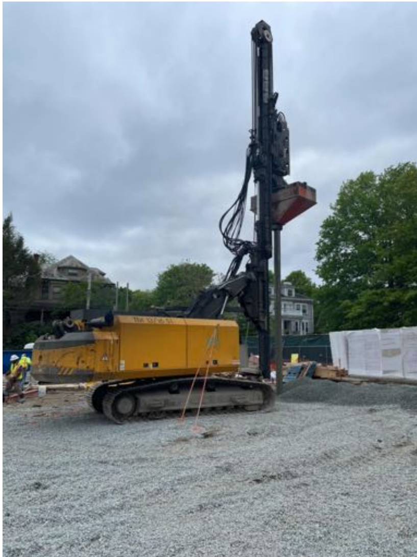
Geopier installation ongoing.
