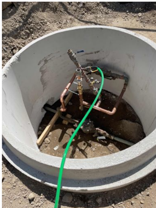
Temporary water service relocated and operational.
