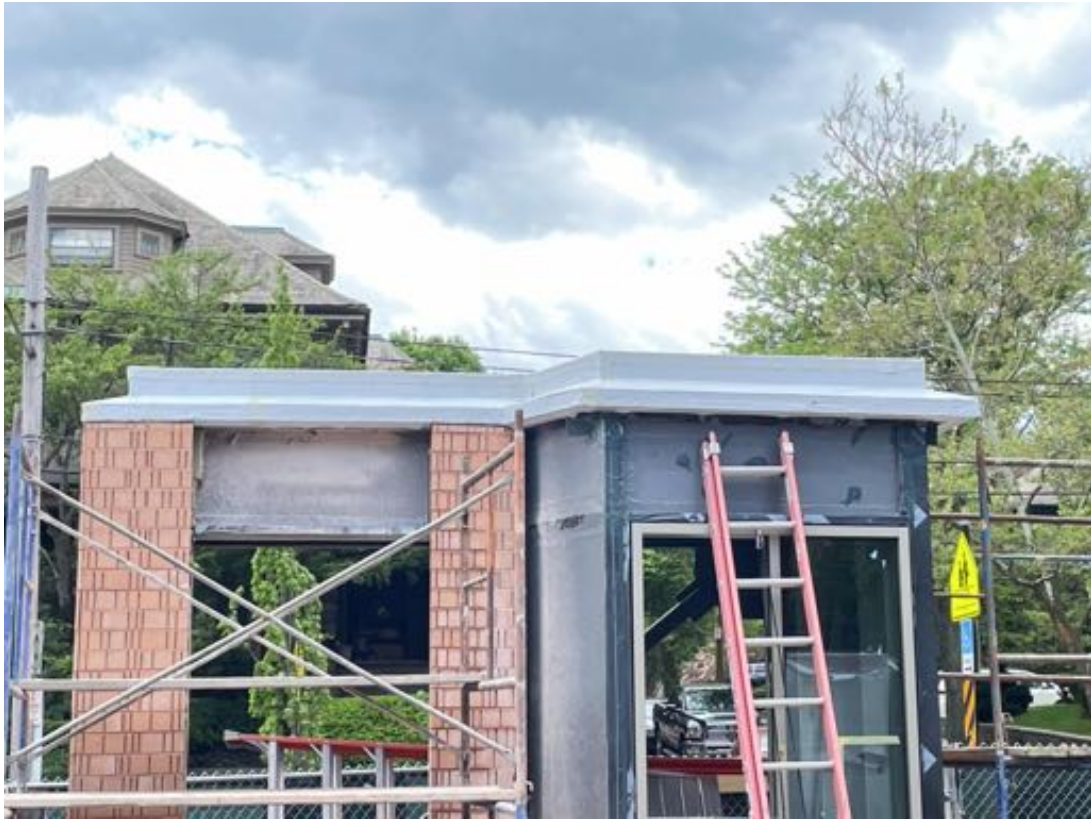
Roofing at mock-up.
