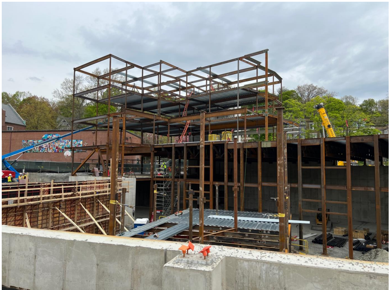
View of steel progress.
