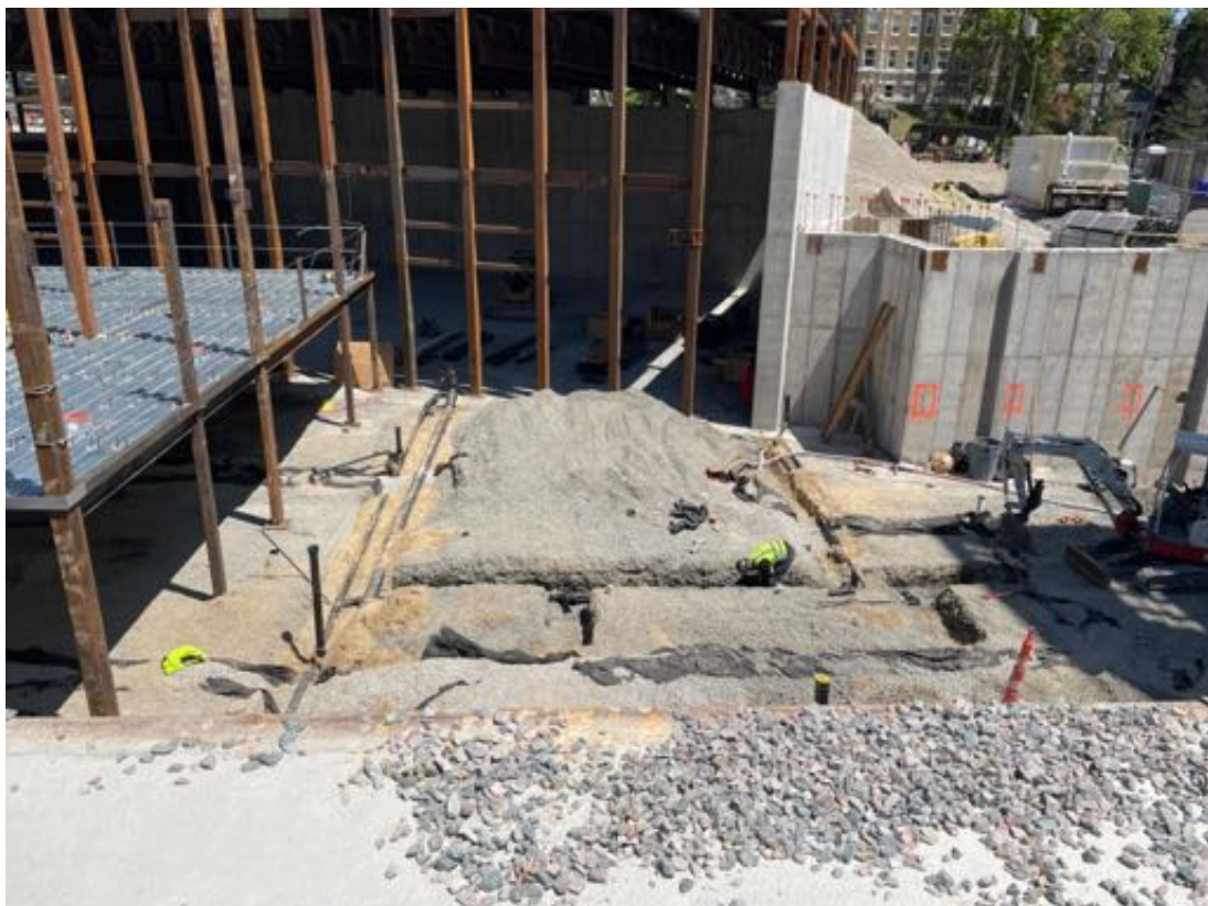
Plumbing backfilled, Area A.
