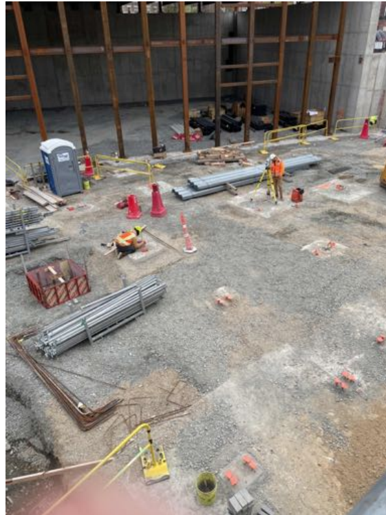
Anchor bolt survey.
