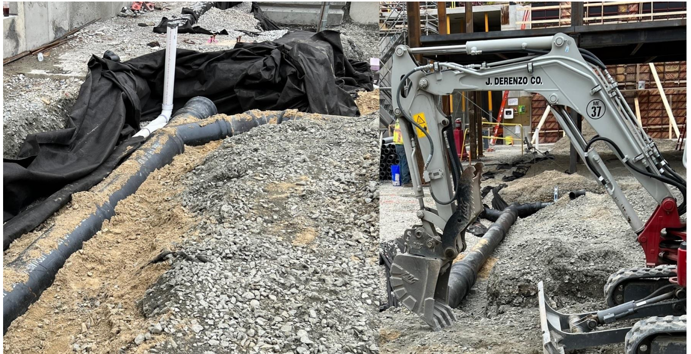
Underground Plumbing in Building C progress.
