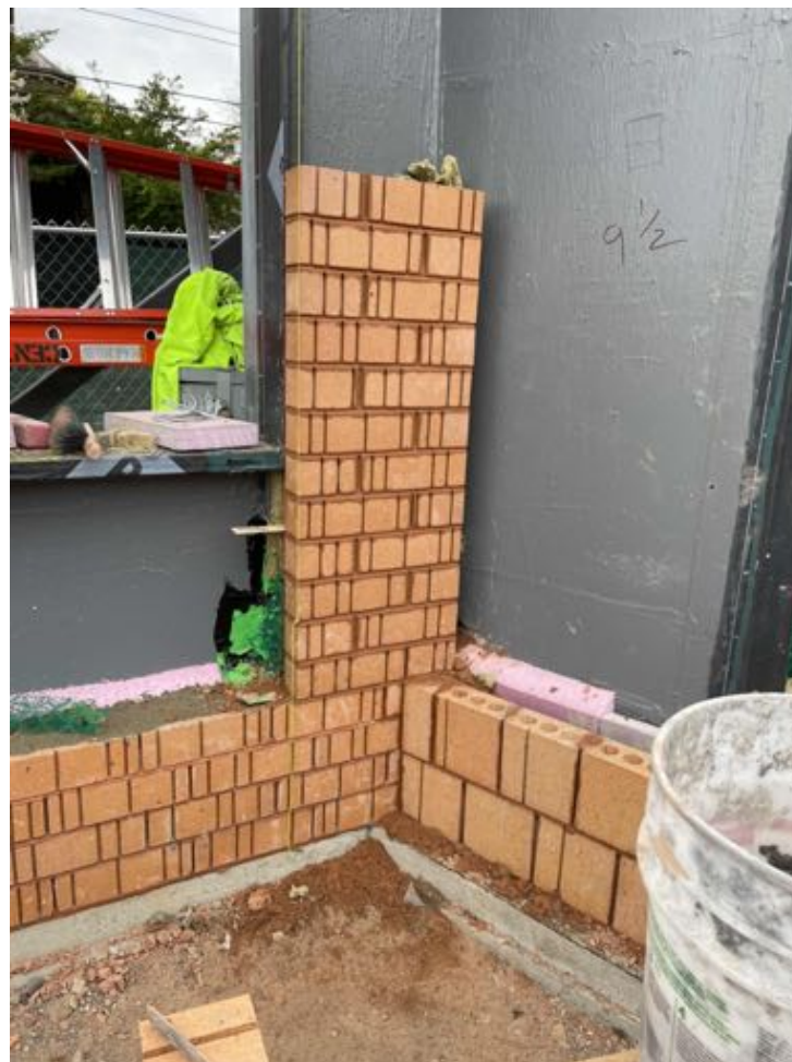
Masonry mock-up.
