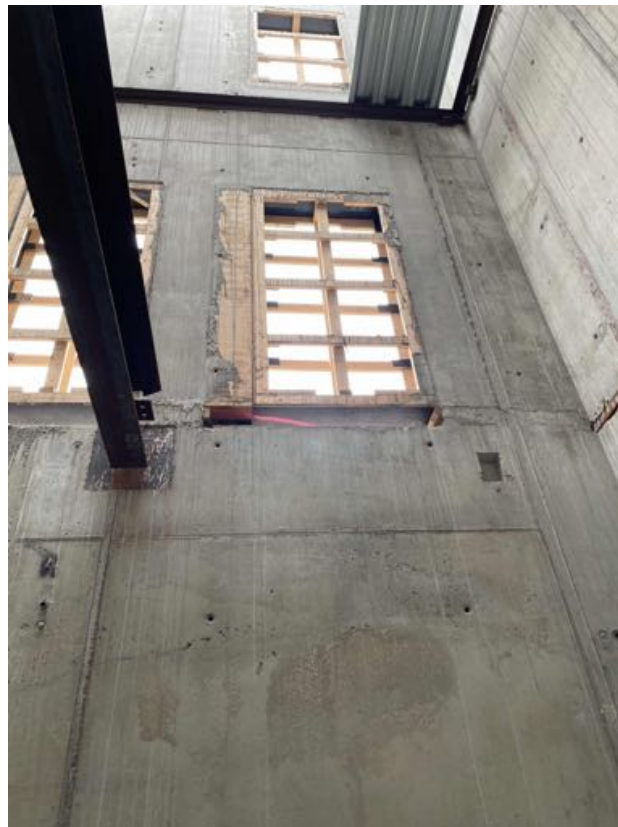
Core C – landing steel and deck.
