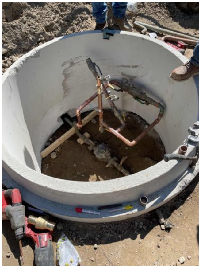
Temp water service relocated along Washington.
