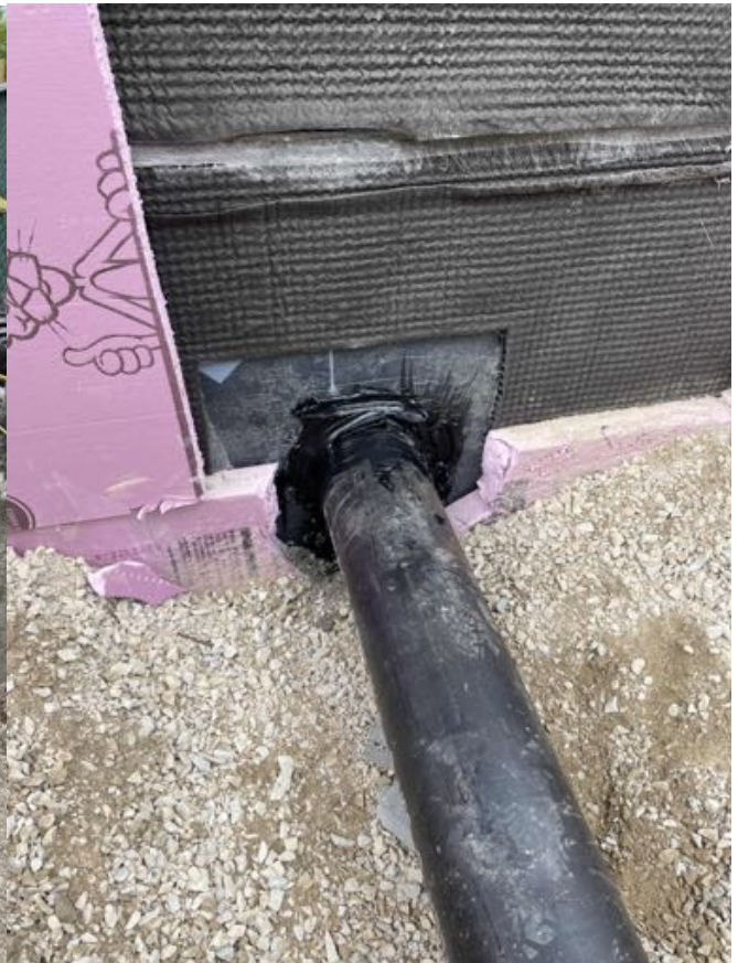
Install plumbing through sleeve, line CY adjacent to existing gym.
