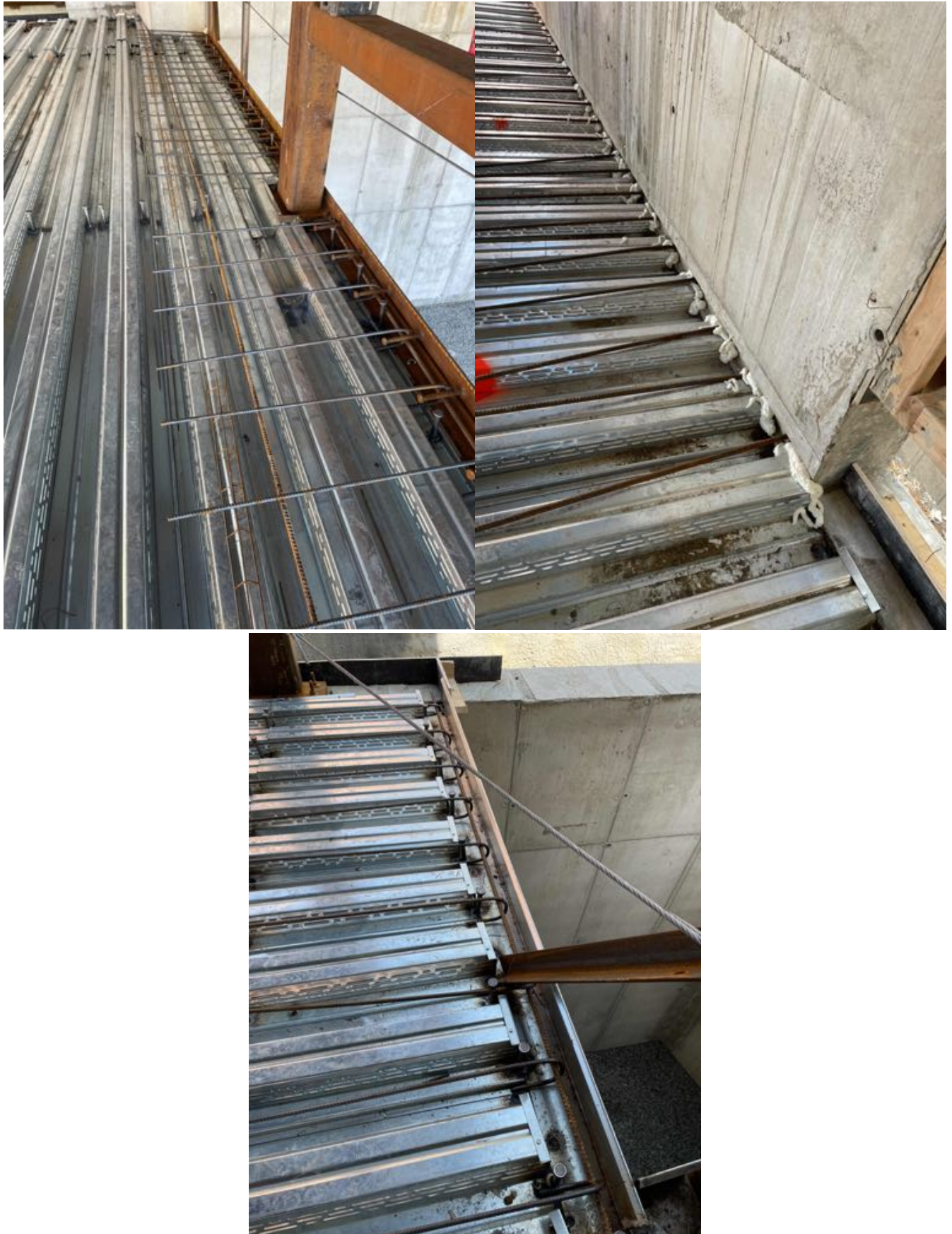
Deck prep prior to concrete pour.
