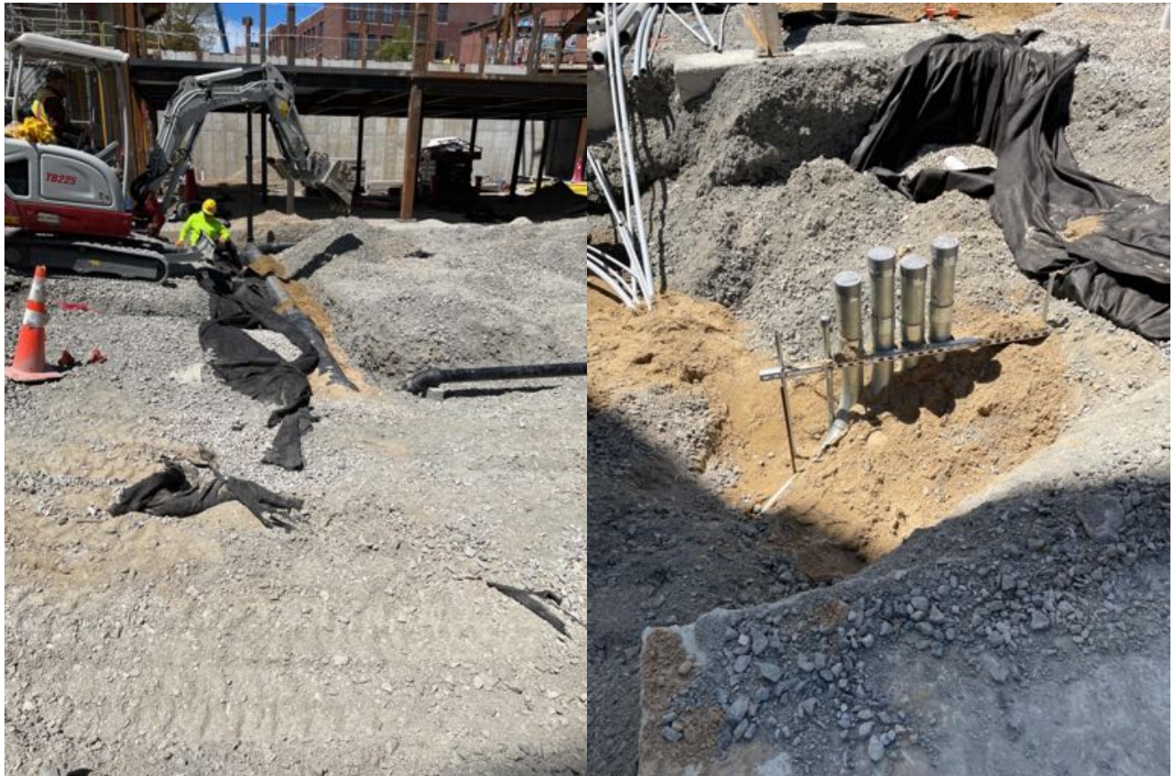
Pipe and conduit progress.
