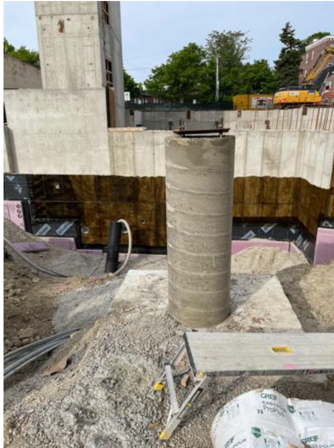
Round column poured and stripped.
