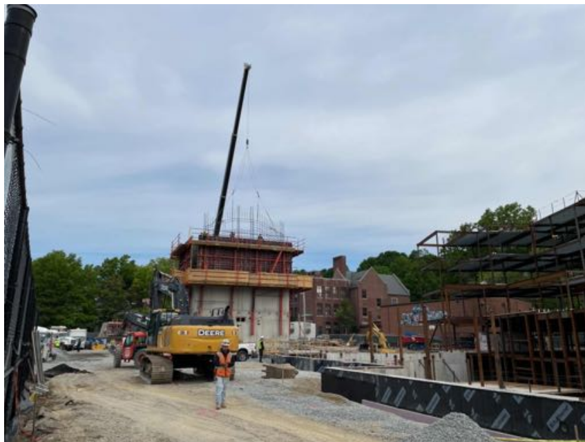
Rebar at Core AB.
