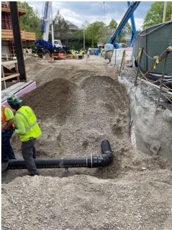
Install plumbing through sleeve, line CY adjacent to existing gym.
