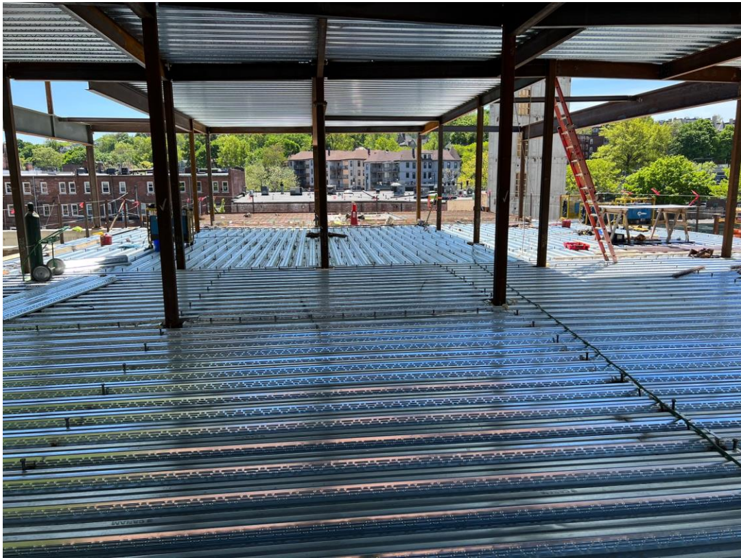
Steel decking/rebar reinforcement on level 2 of Building C.
