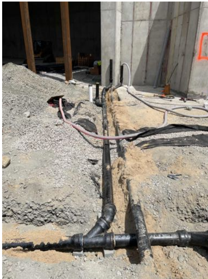
Underground plumbing progress.
