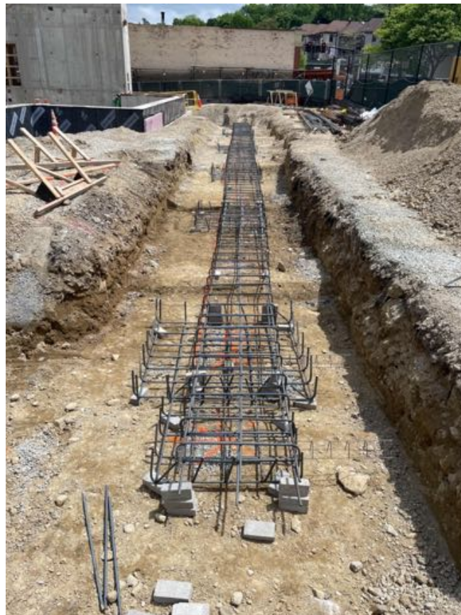
Rebar at footings along line AD.
