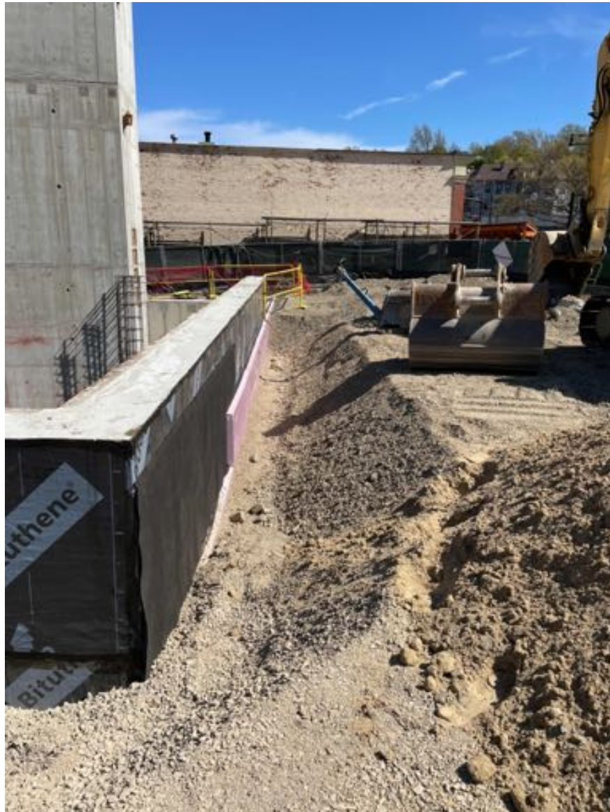
Backfill along Washington St.
