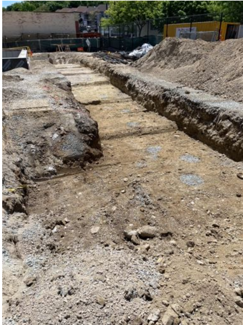
Excavation for footings at geopiers, line AD.
