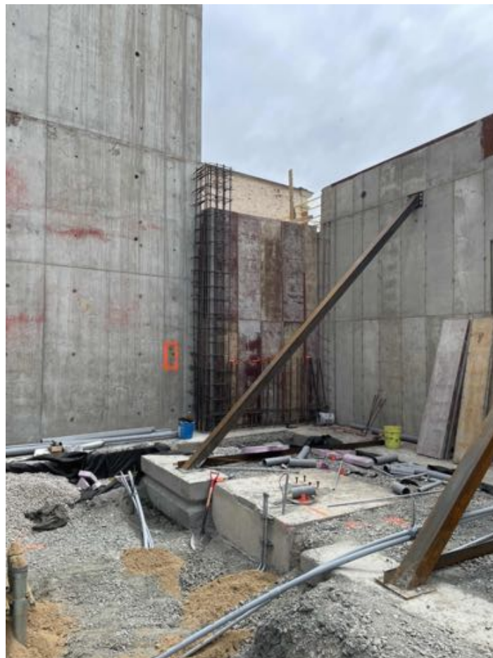
Forms and rebar at areaway, SE.
