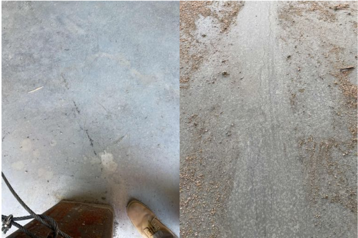
Slight crack in floor slab C1.
