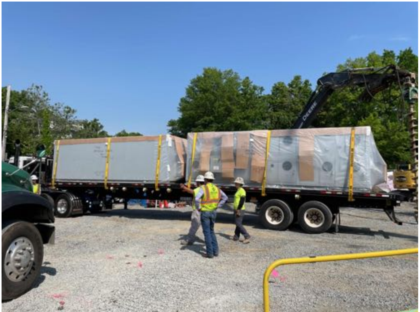
Air Handling Units (AHUs) arriving on site.
