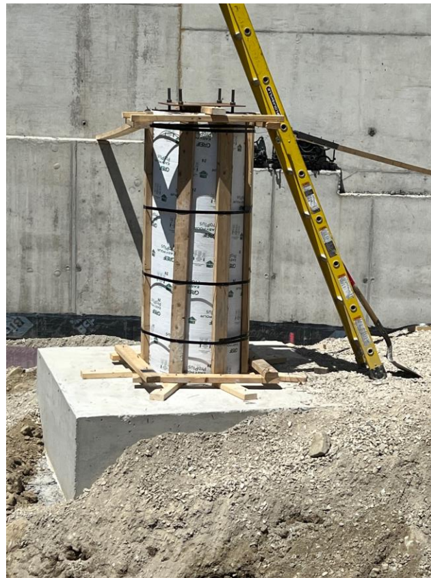
Forming for Column at line AX (loading dock)
