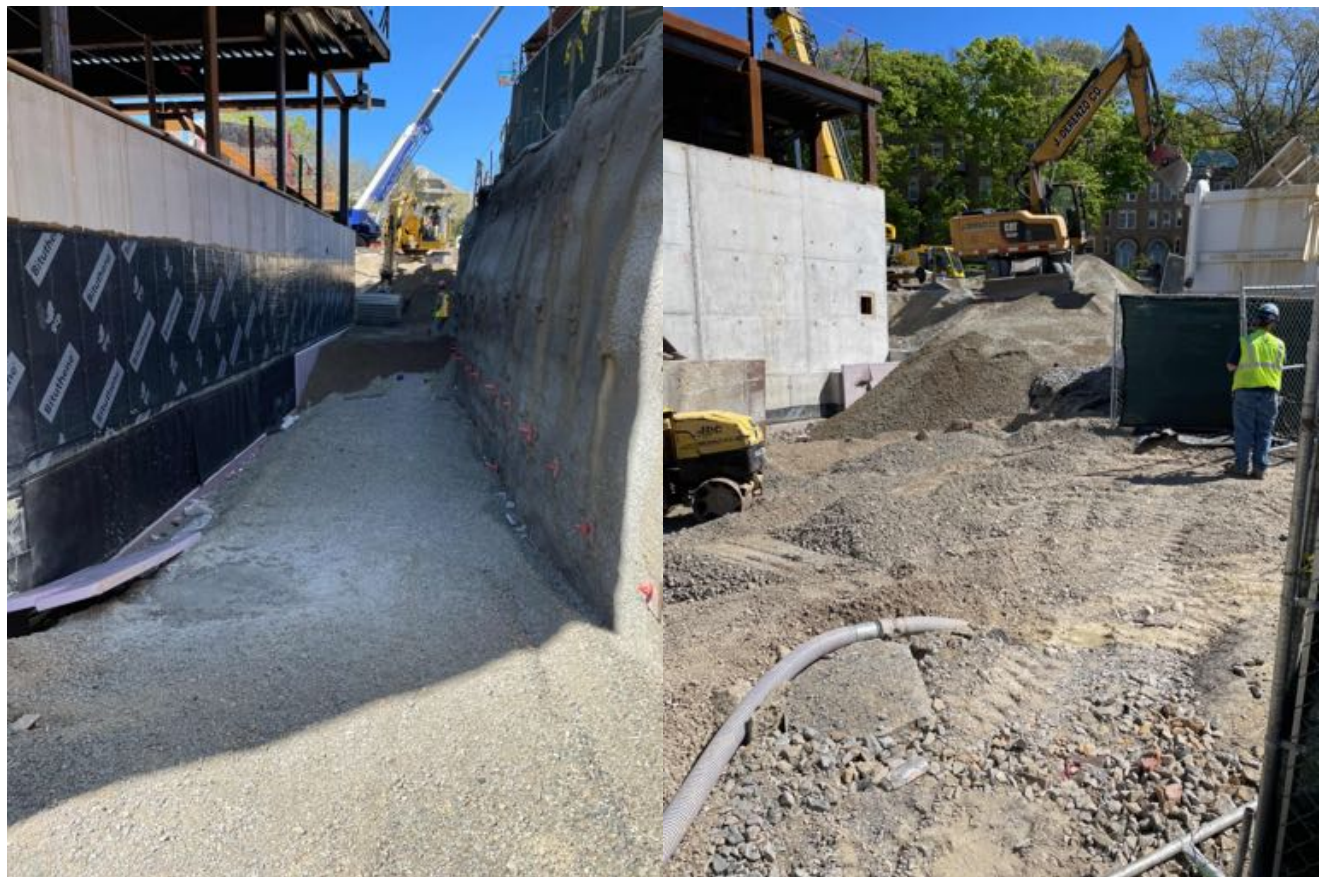
Backfilling.
