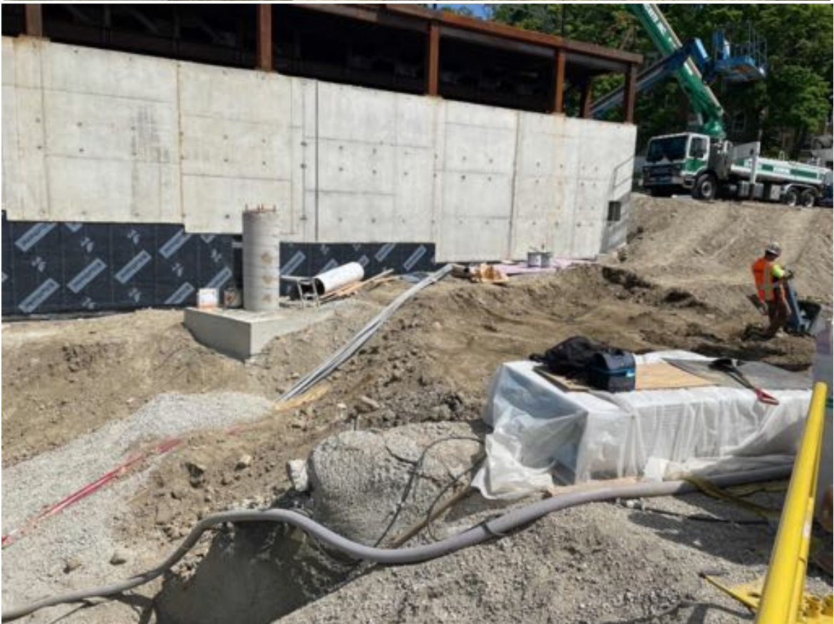
Waterproofing, backfill and compaction at ductbank.
