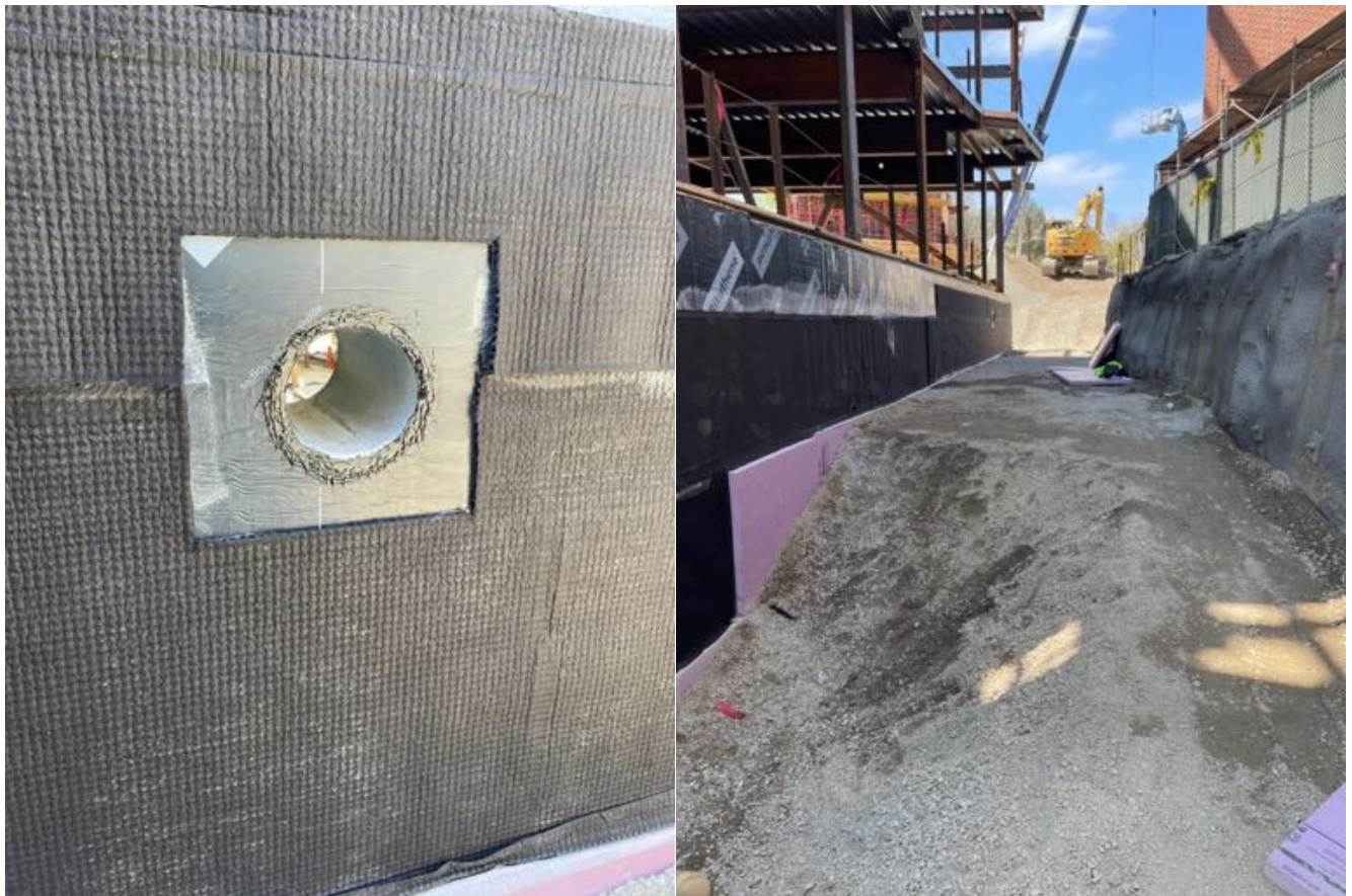
Backfill and waterproof wall CY.
