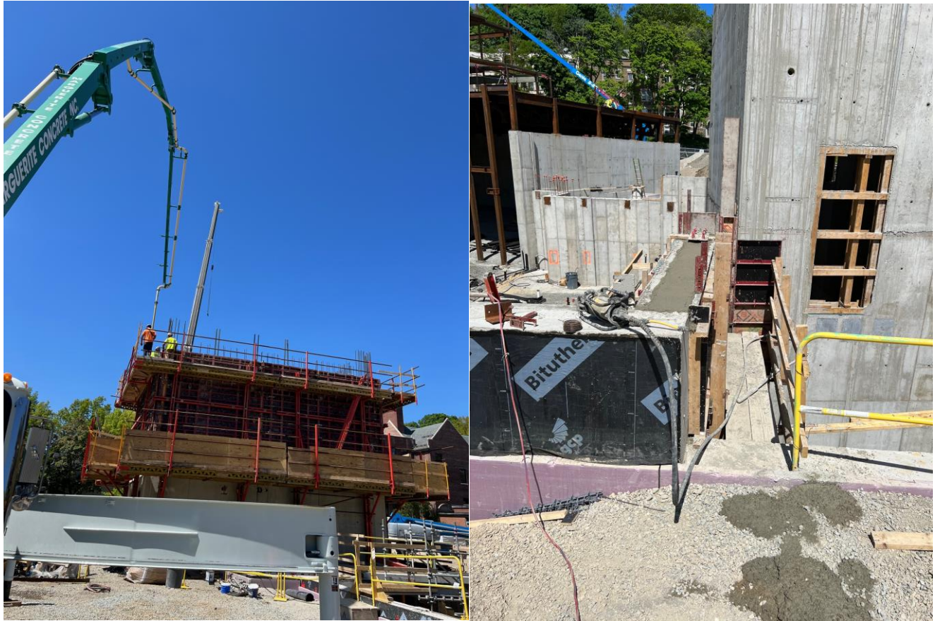
Concrete pour at Core AB level 2, and generator areaway
