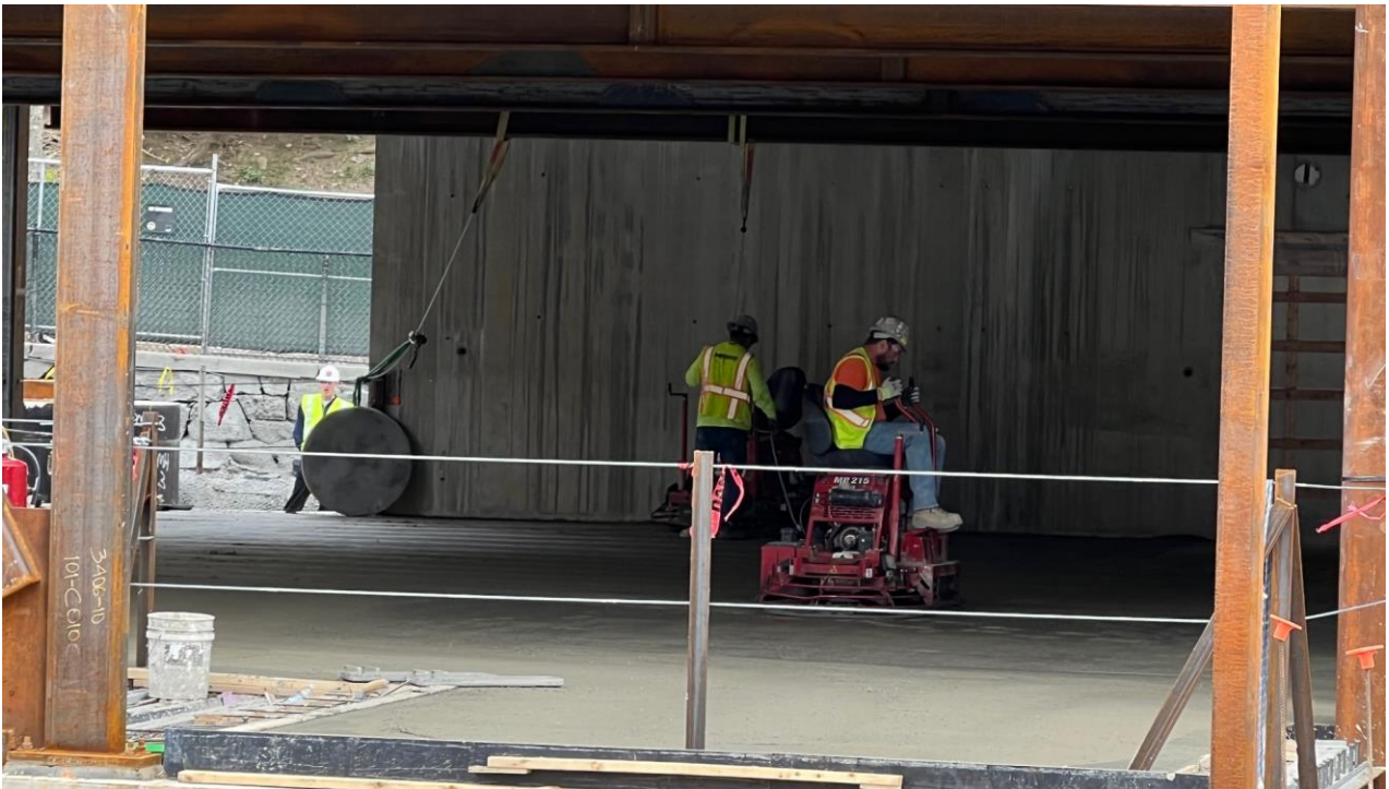
Finishing underway on deck slab C1.
