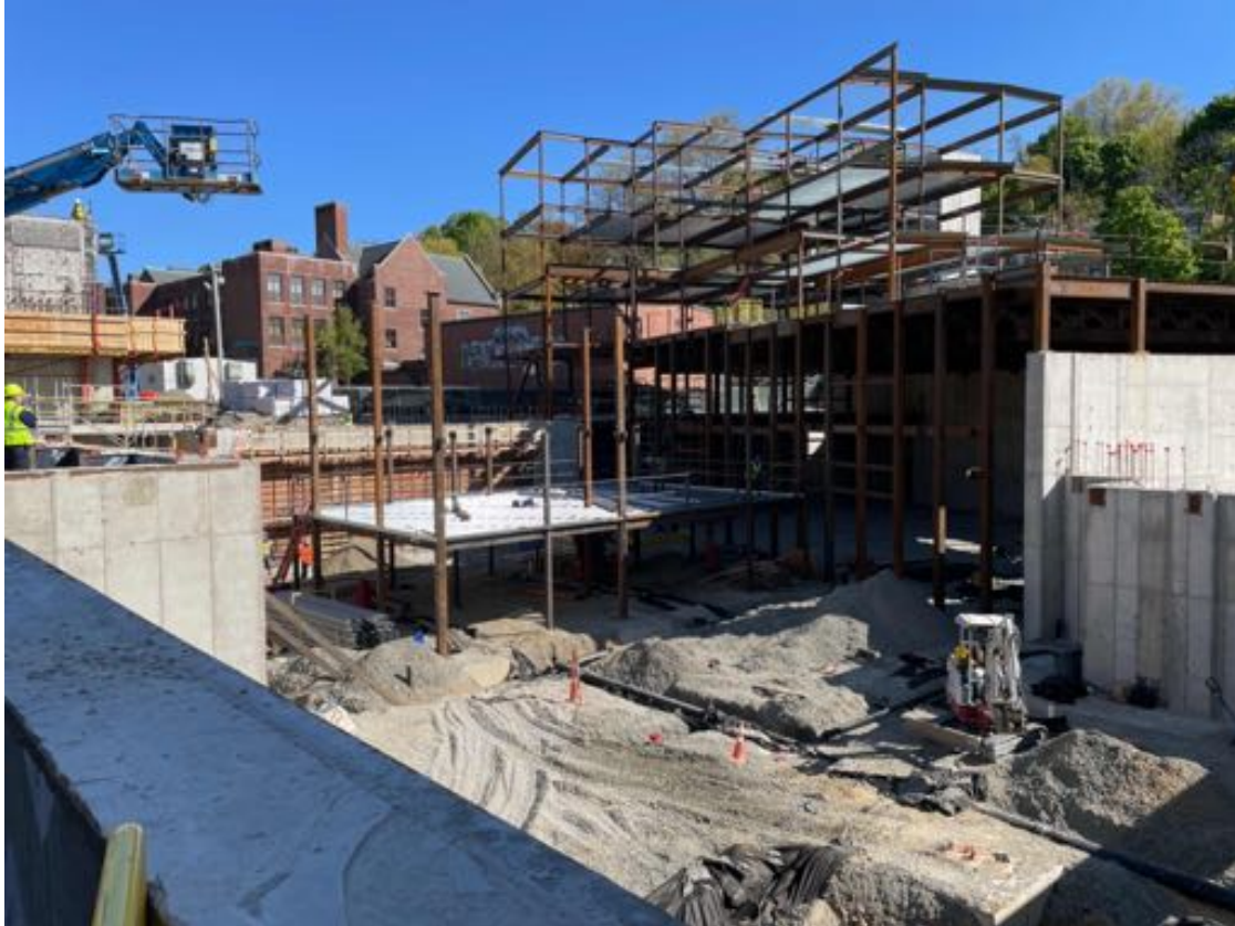
Mezzanine decking complete.
