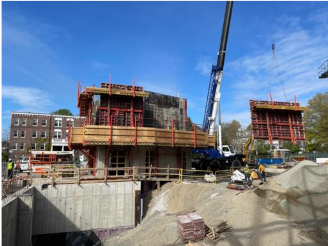
Core AB forms ongoing.
