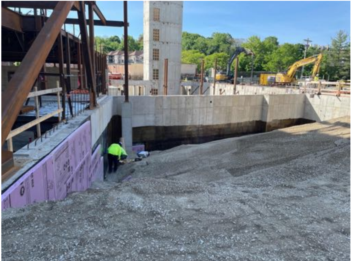
Waterproofing at line A1.
