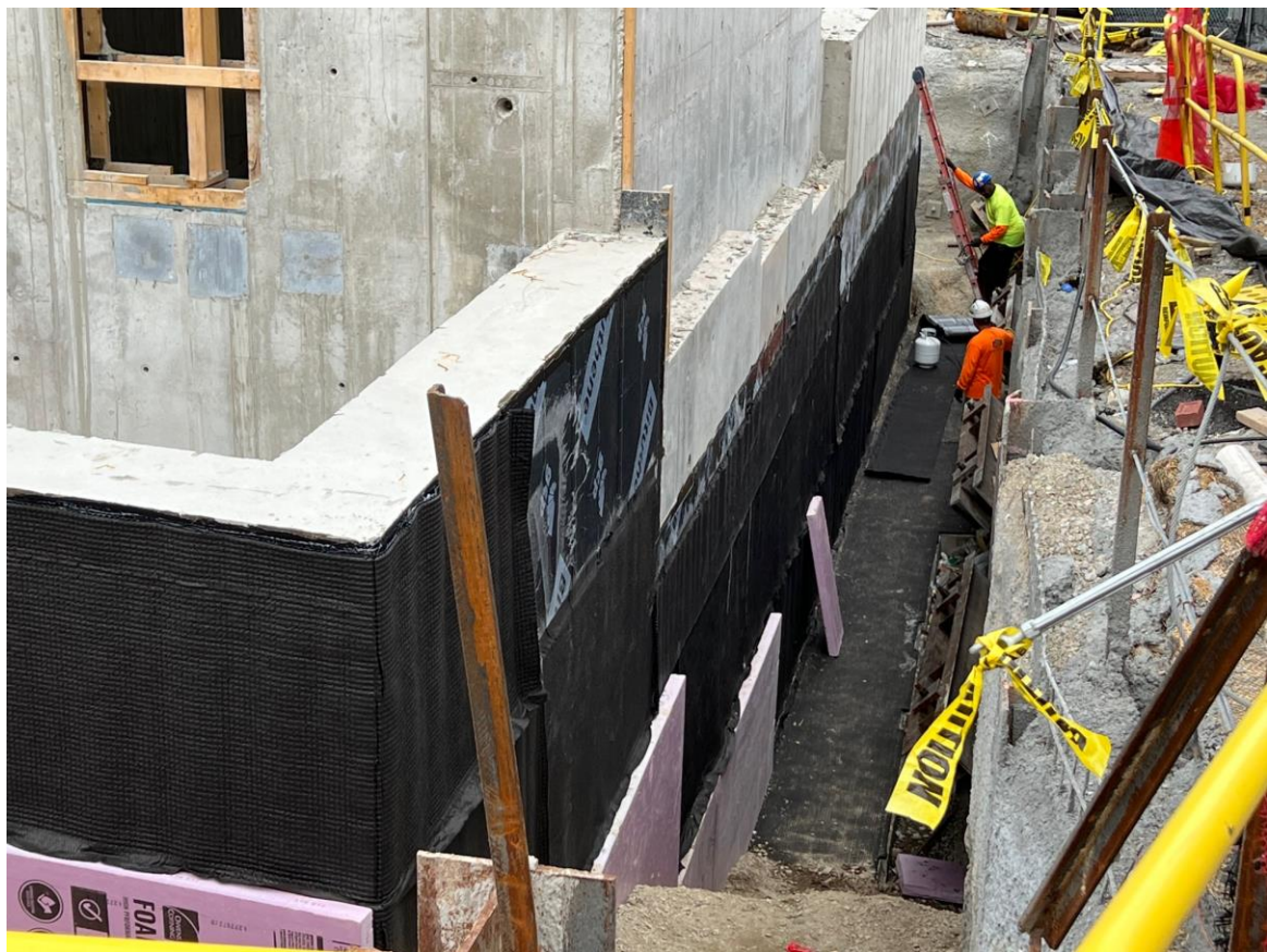
Waterproofing behind Core A (corner of washington st & alleyway)
