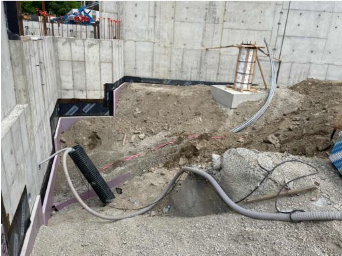
Backfill at utility corridor.
