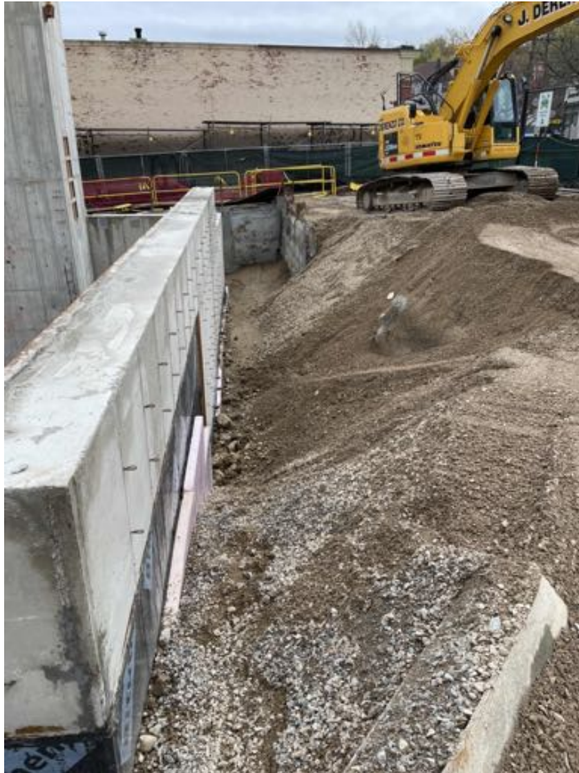
AG near Core A backfilled.
