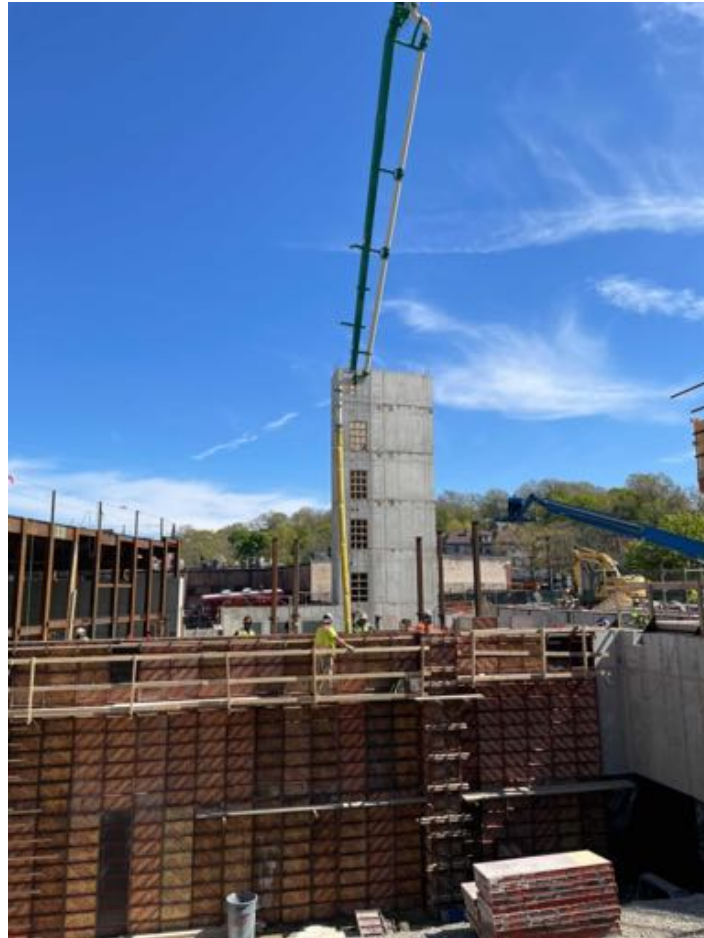
Concrete pour, wall at A1.
