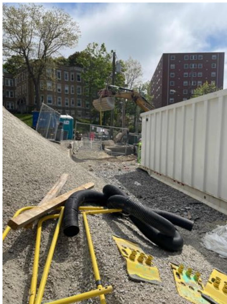
Frac tank #1 removed.
