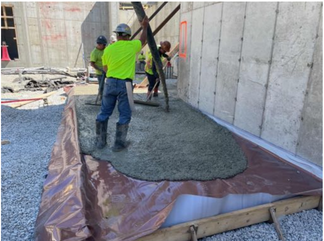
Slab on grade (SOG) poured.
