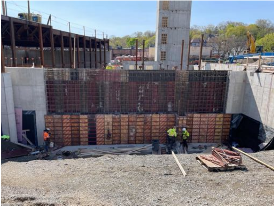
Foundation wall forms at A1.
