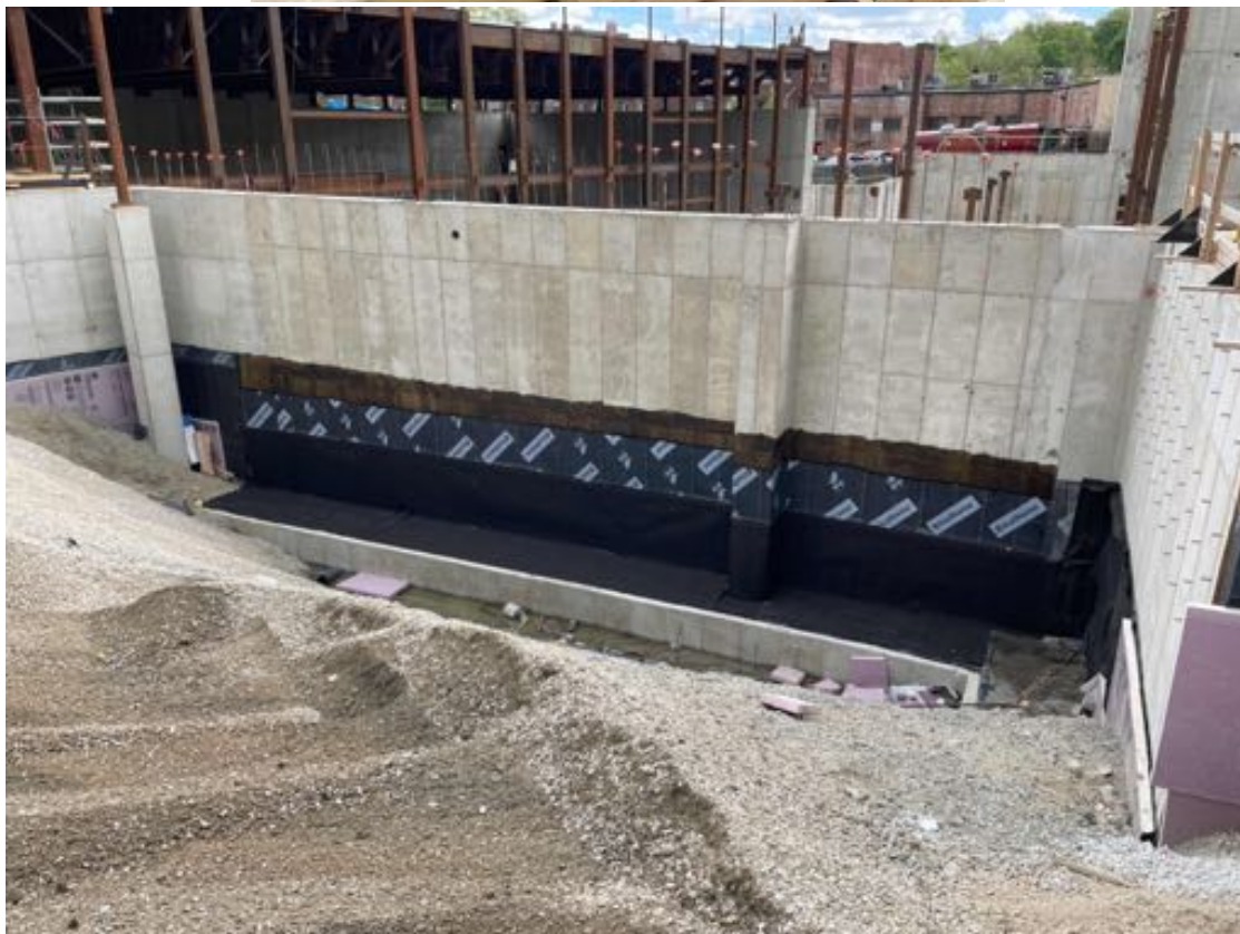
Waterproofing at line A1.
