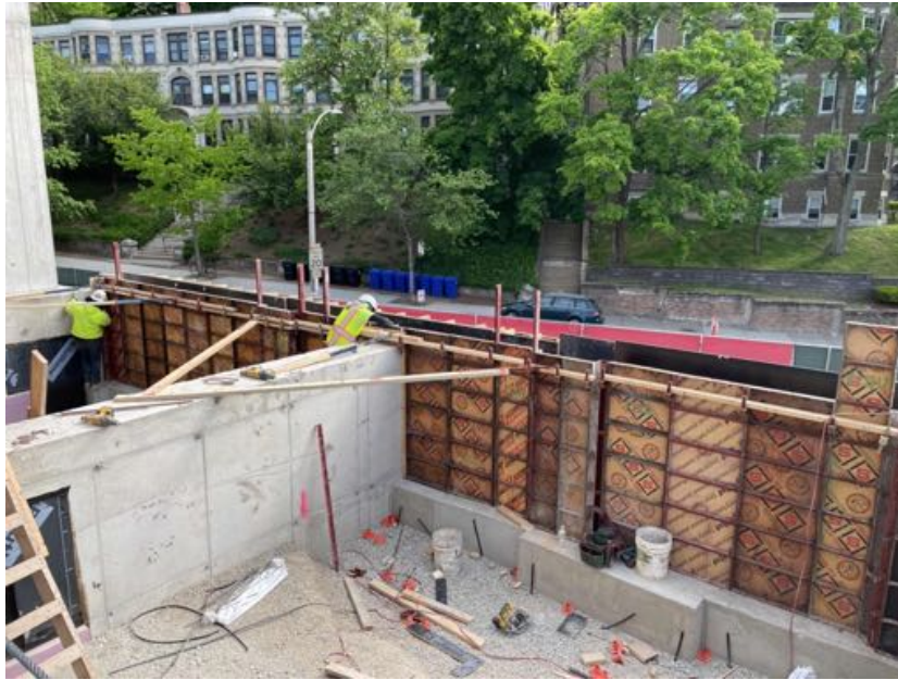
Forms at line C25
