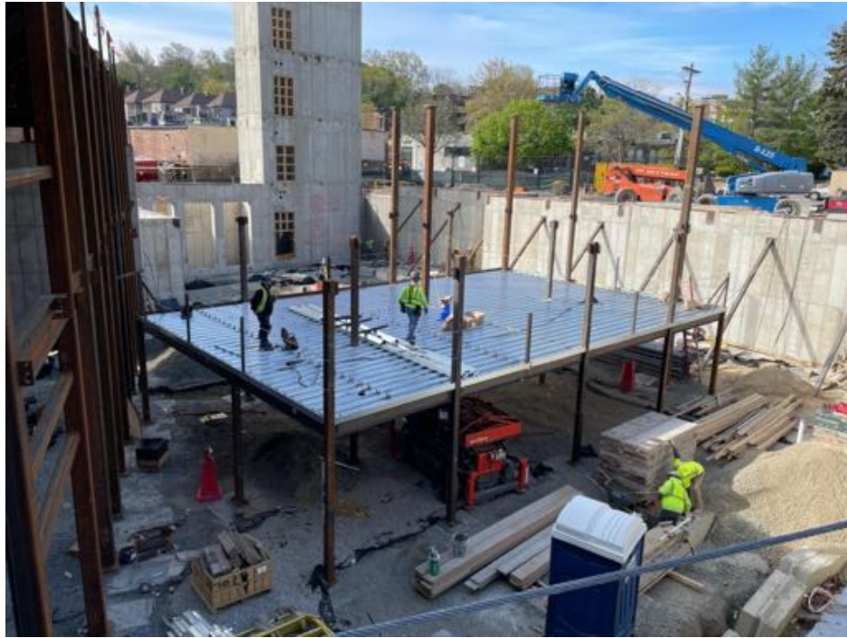
Welding studs at mezzanine.
