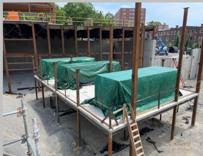
AHU in place at Mezzanine Level
