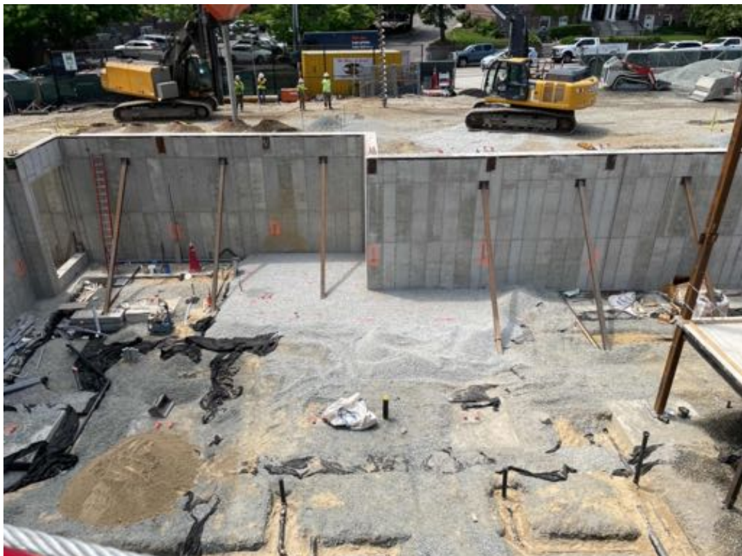
Prep for slab on grade at generator.
