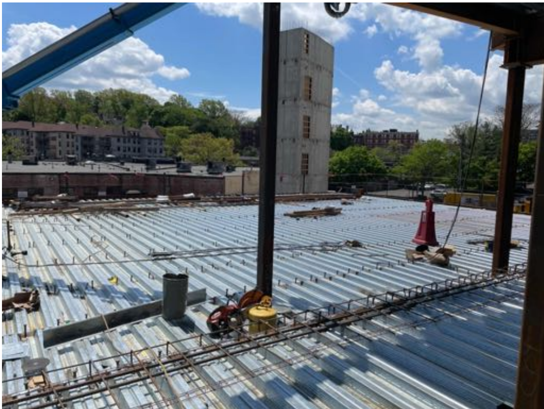
Steel decking/reinforcement at Level 2.
