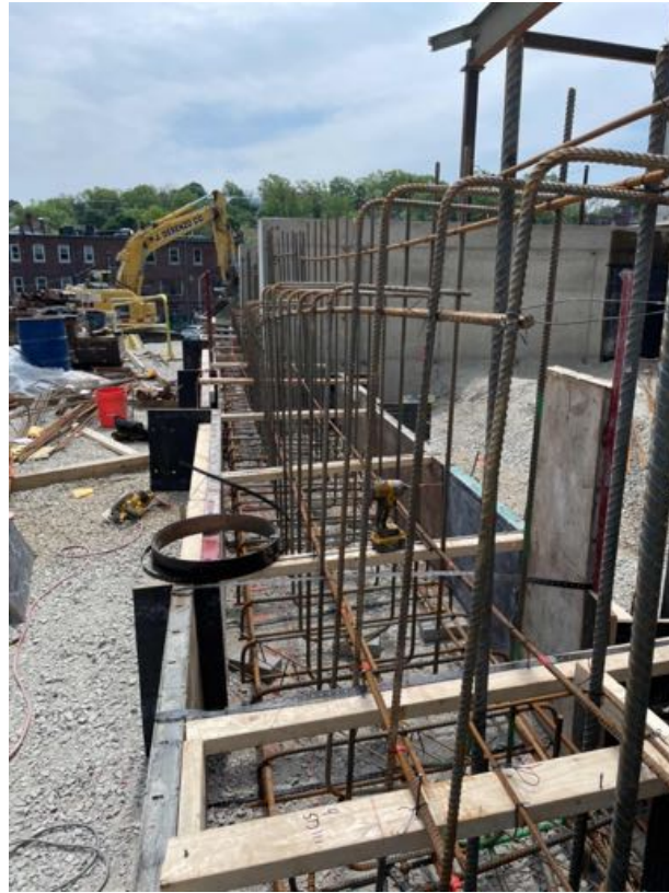
Footings at North side.
