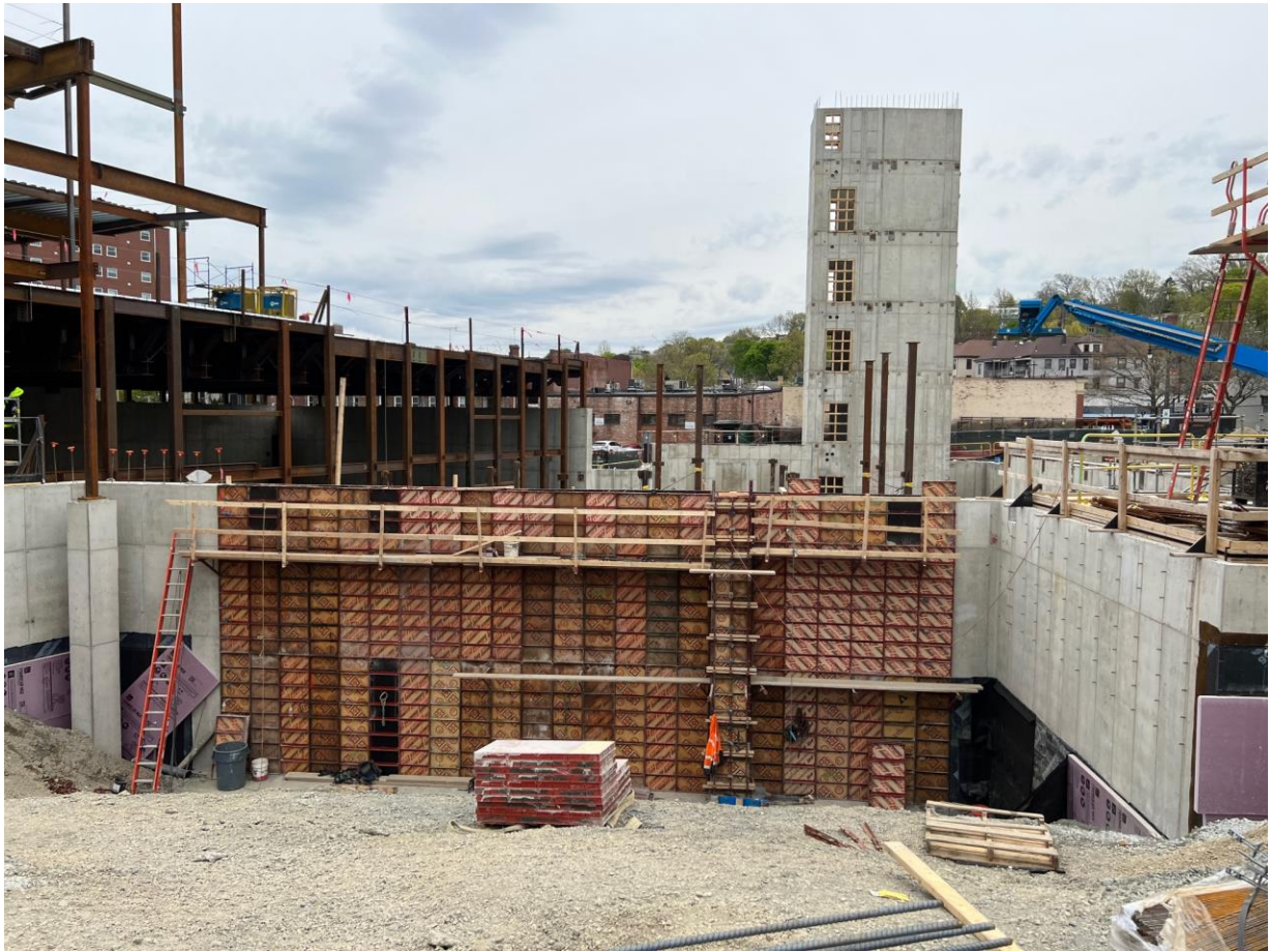
Foundation wall forms at A1 prepared for Monday's pour.
