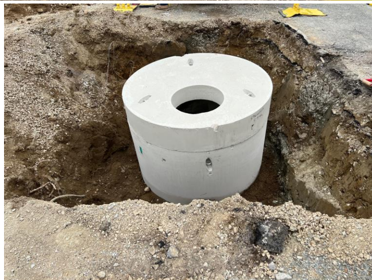
Water service work along Washington St.
