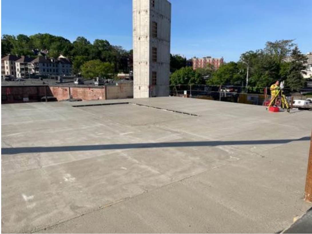
Slab at C2 completed. Flatness test performed by UTS.
