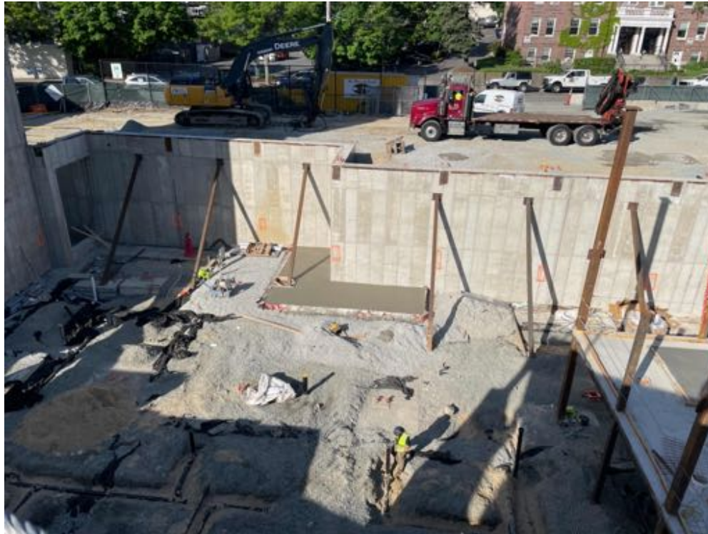
Slab on grade at generator completed.
