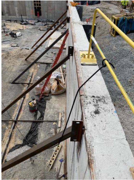
Clips welded along line AG.
