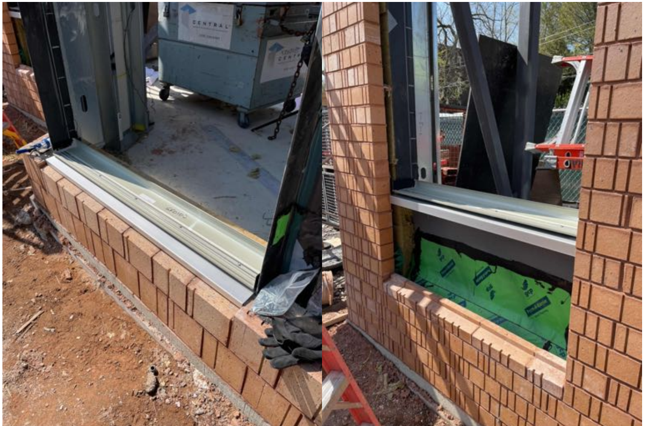
Window frames at mock-up.
