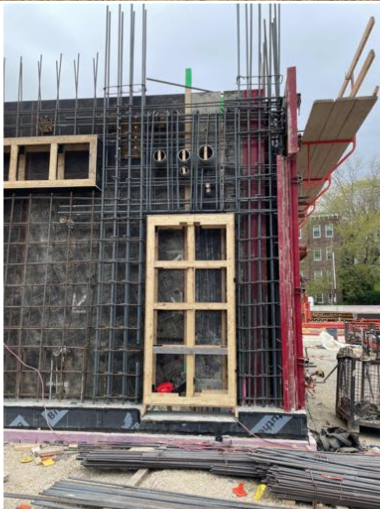
Setting forms, rebar and embeds, Core AB.
