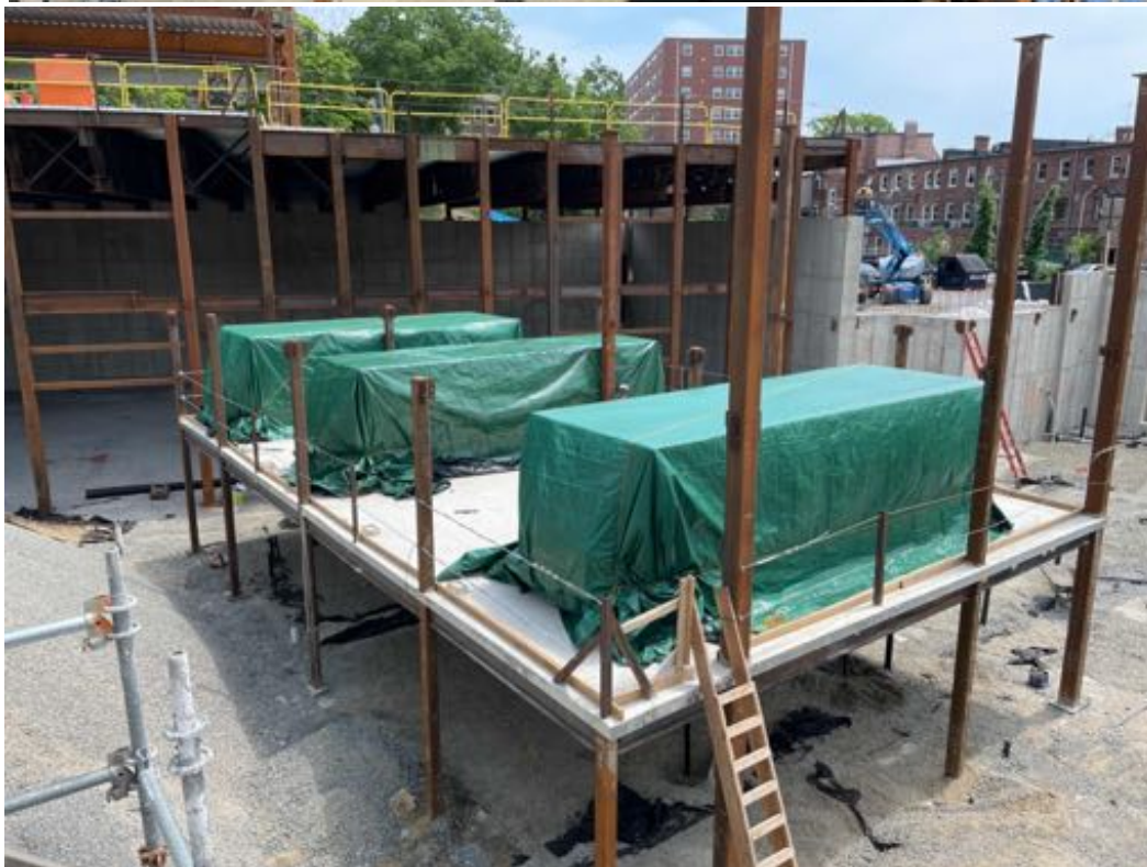
AHUs in place on mechanical level.
