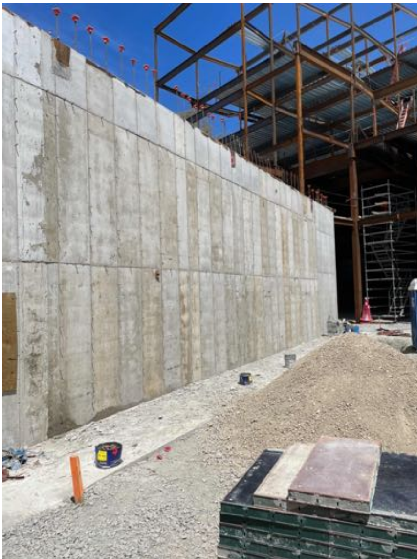
Wall at A1 stripped.
