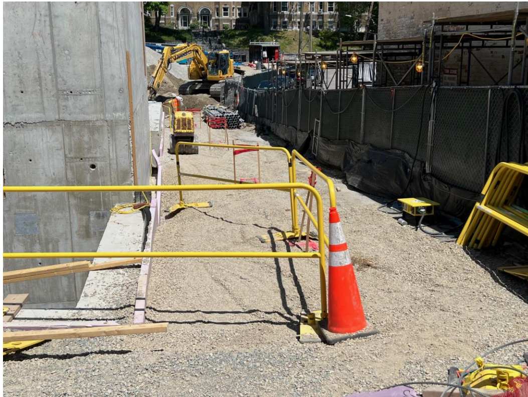
Backfill and Compaction behind Core A
