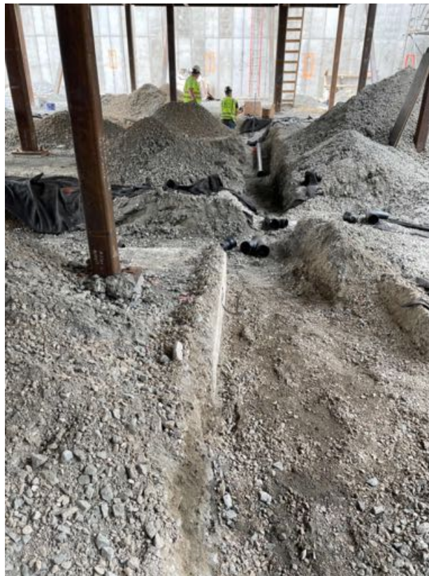
Plumbing excavation, toilets rooms under mezzanine.
