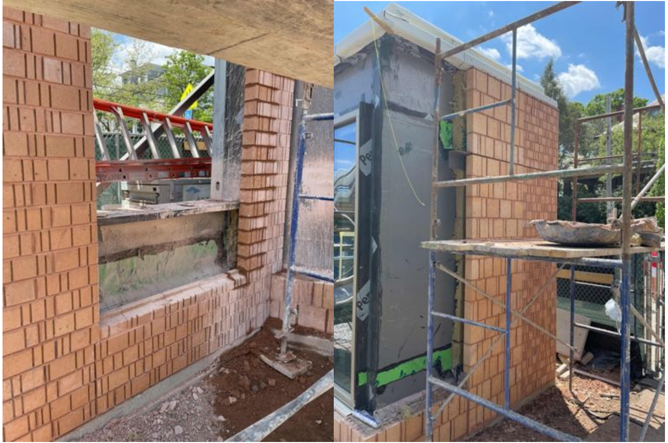
Masonry at mock-up.
