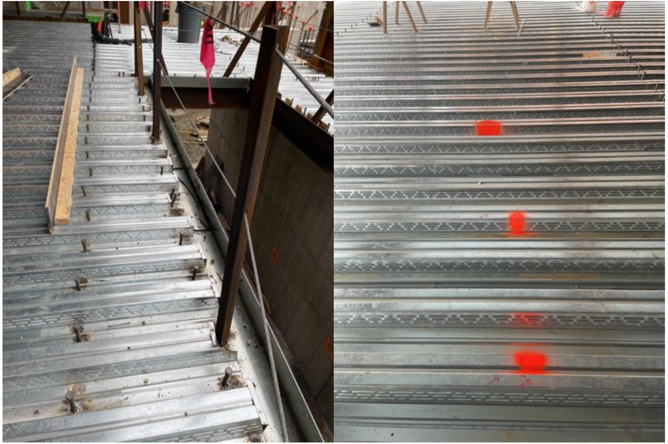
Deck at CY/CT.8, Level 2.
