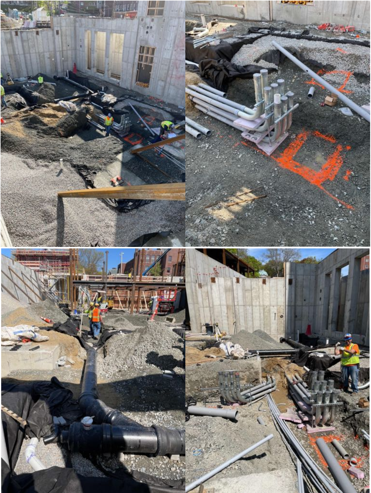
Underground pipe progress.
