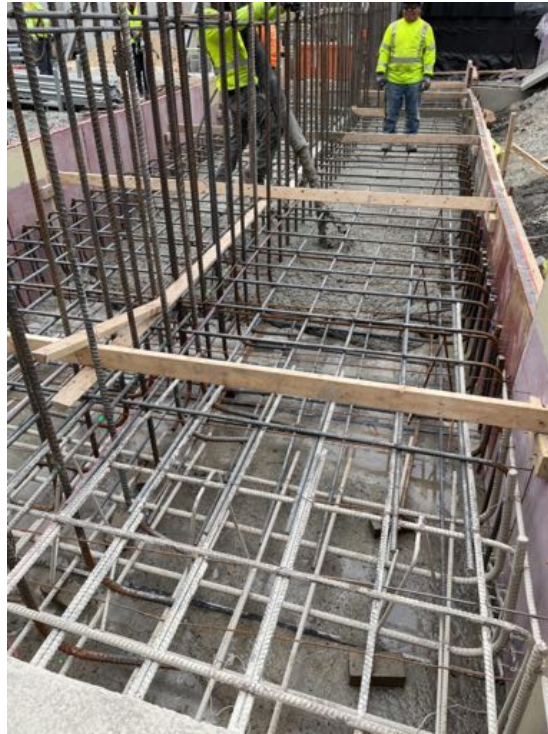
Footing at A1 – concrete pour.
