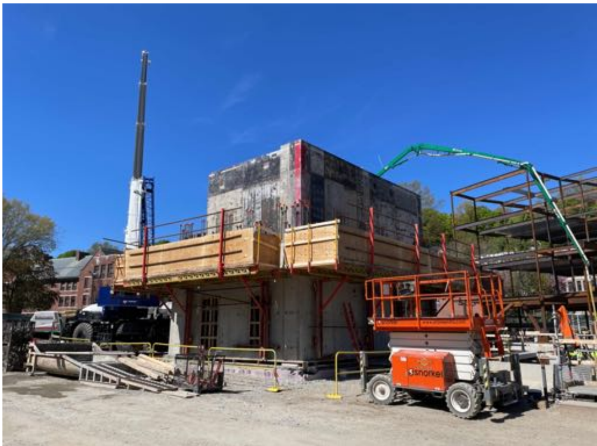
Form installation at Core AB.
