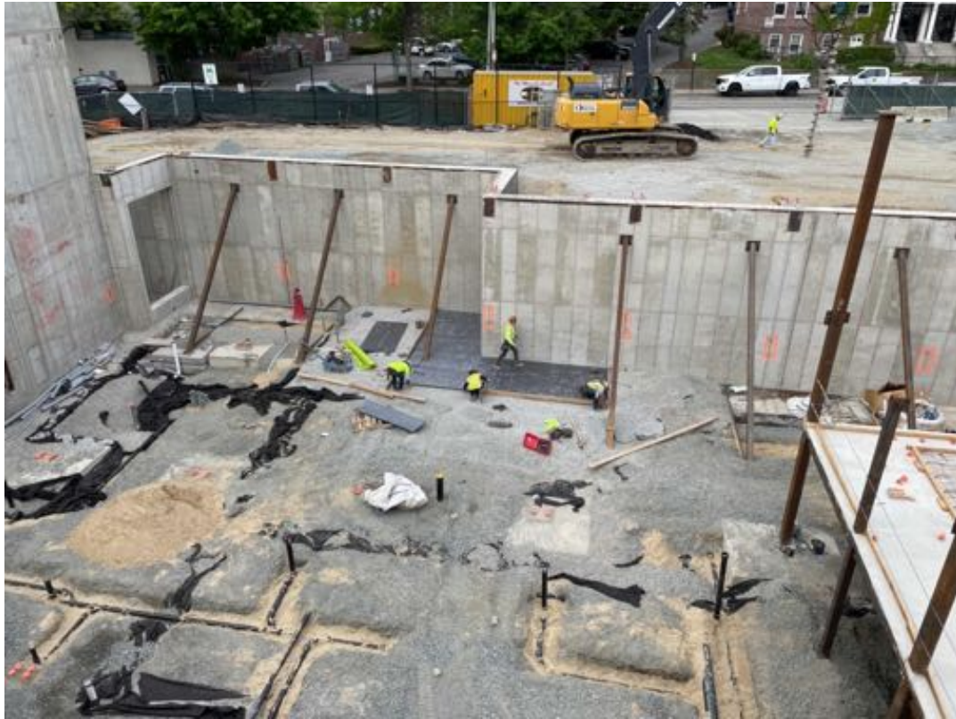
Slab on grade prep.
