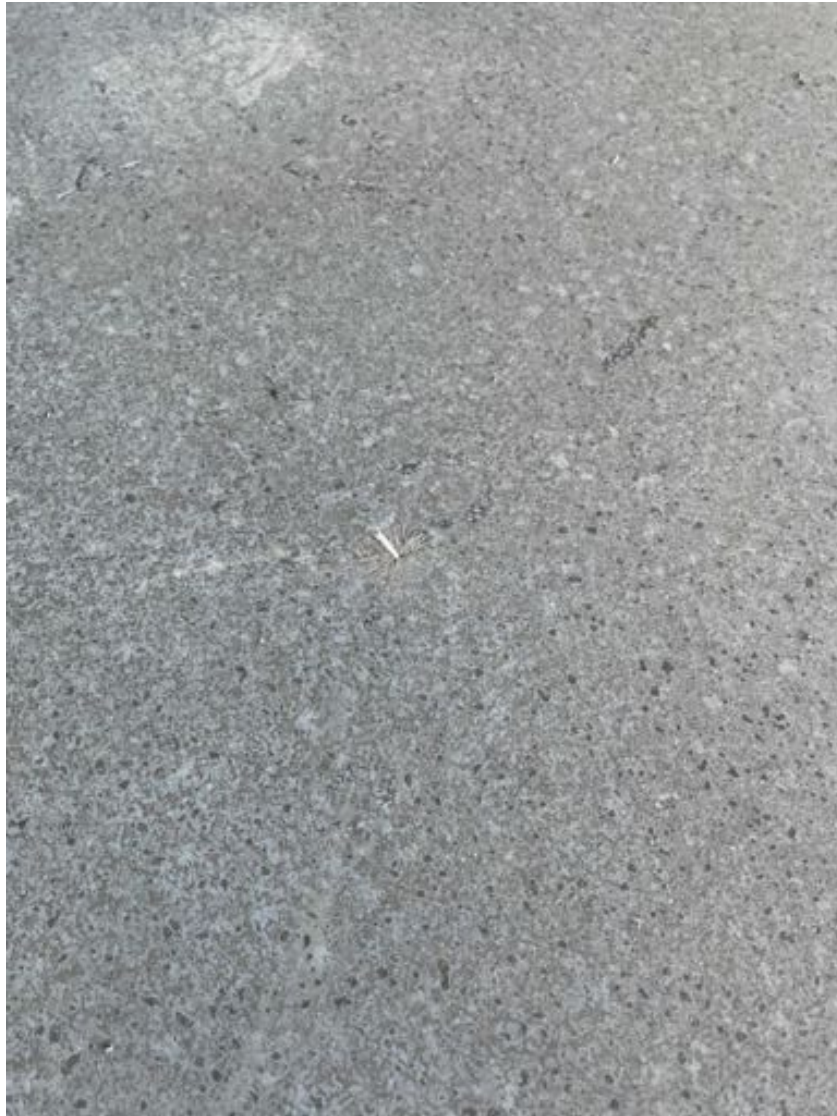
Fiber in slab, very limited.
