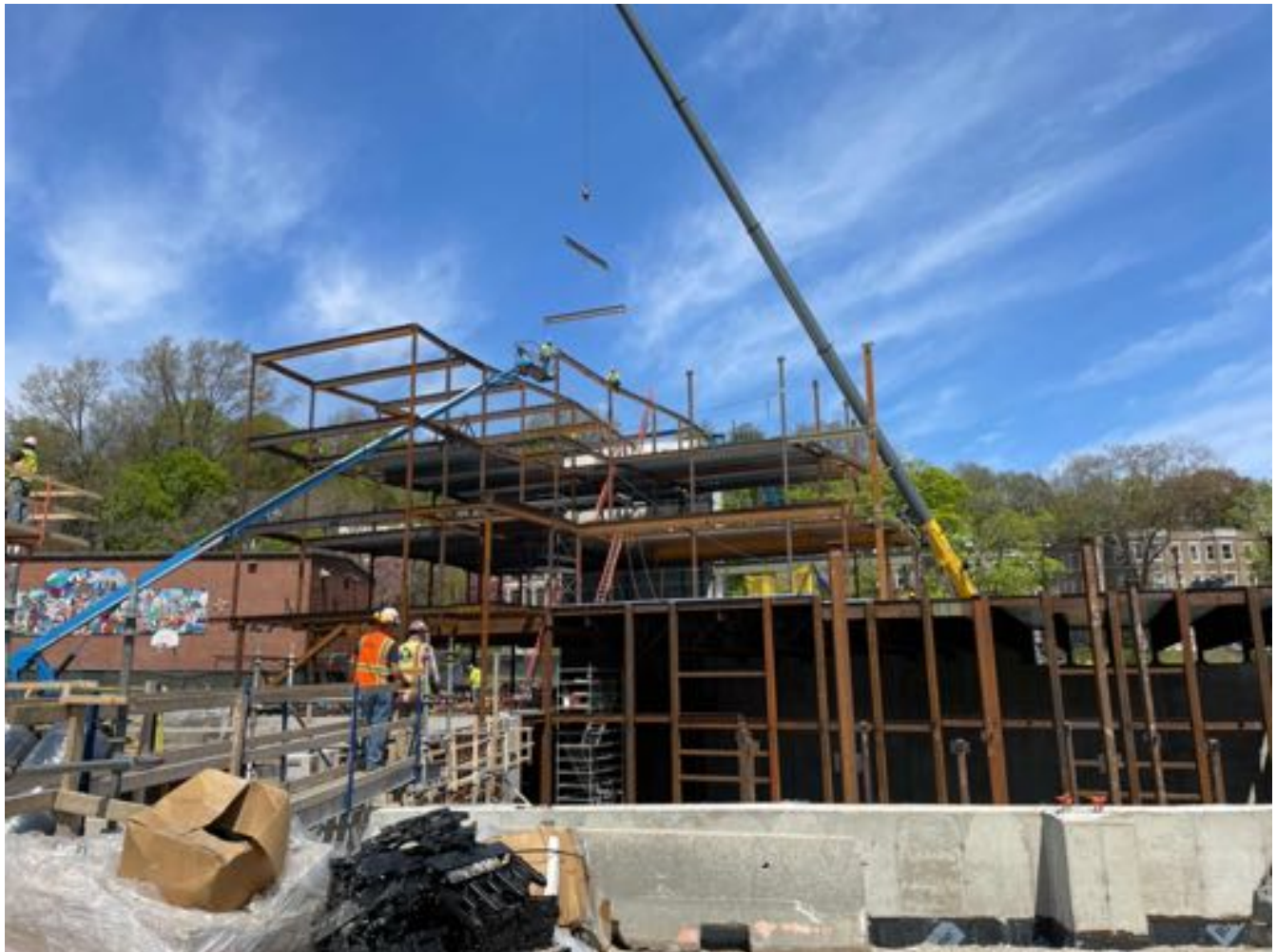
View of steel.
