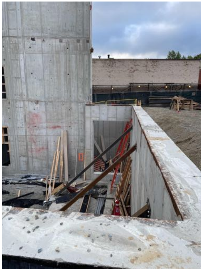
Generator areaway forms stripped.
