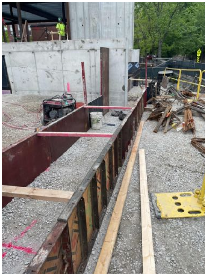
Forms for footings at North side.
