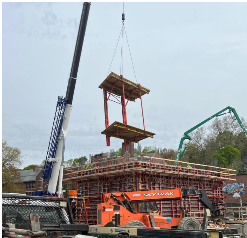
Forms being installed at Core AB level 2
