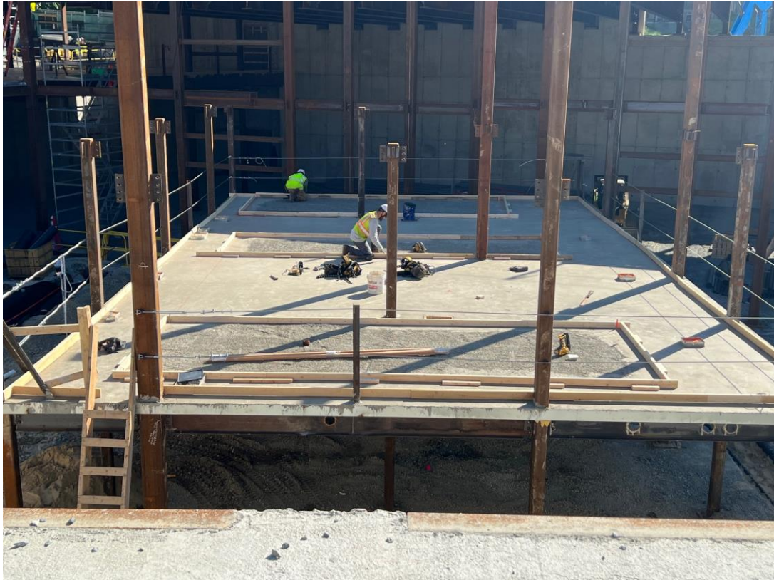
Prepping mezzanine for installation of housekeeping pads.
