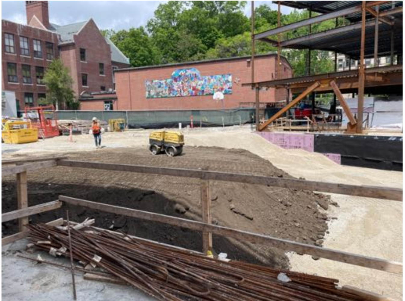
Backfill and compaction along A1.
