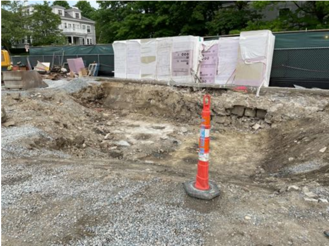
Excavation for mat slab at Core B
