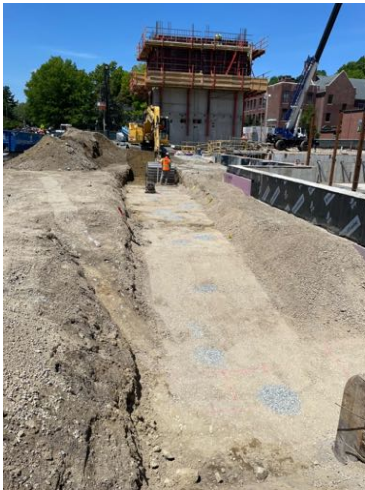
Footing prep along line AD (Washington St.)
