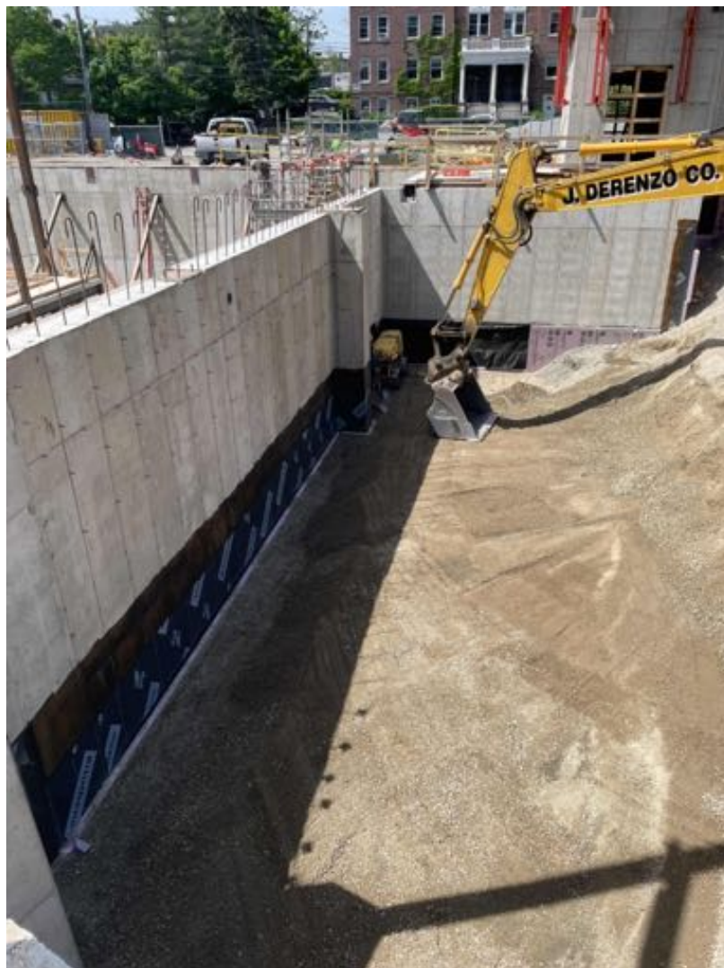
Backfill and compaction at line A1
