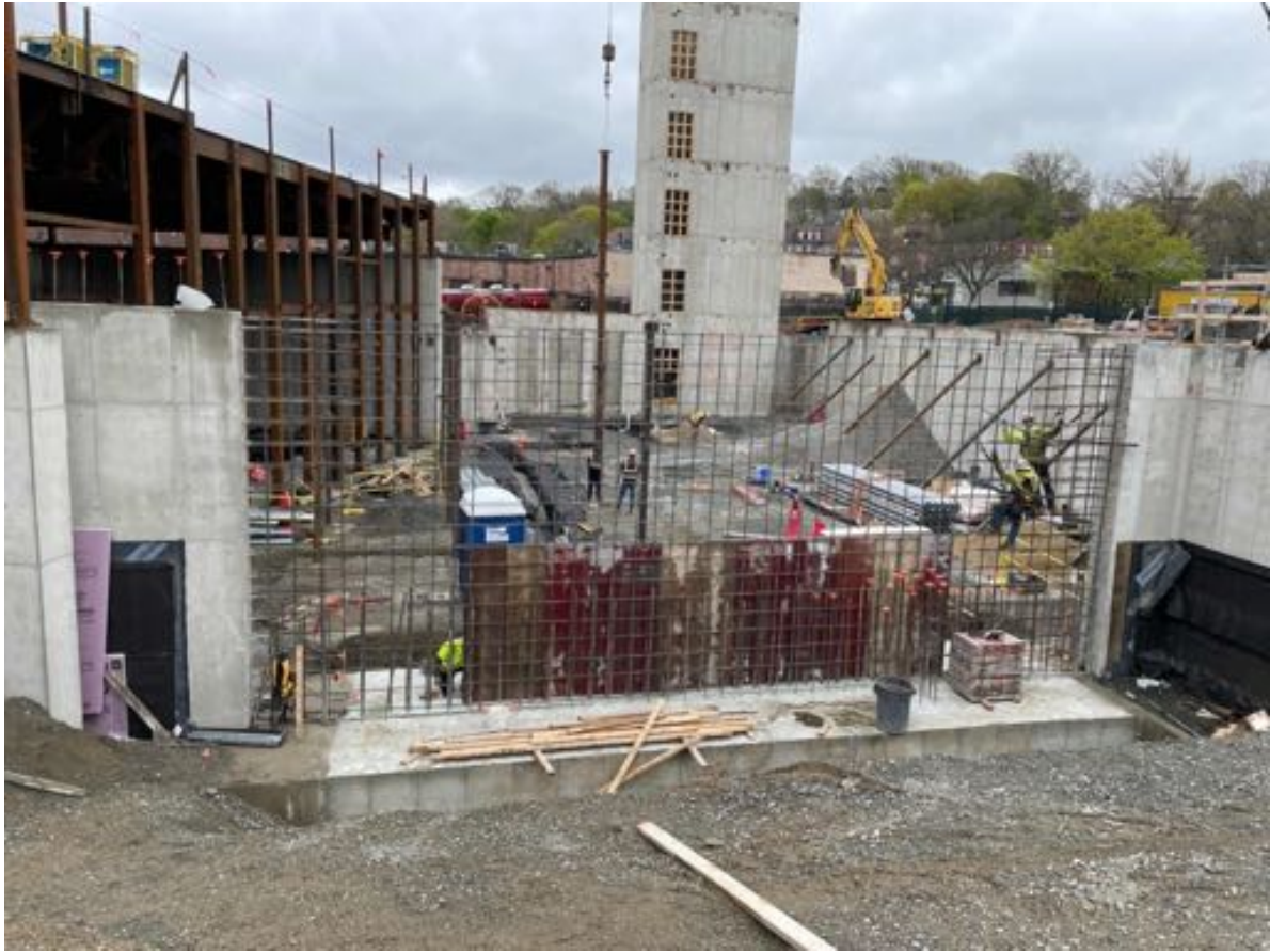
Rebar and forms for wall at A1
