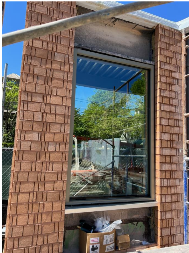
Window installed at mock up.
