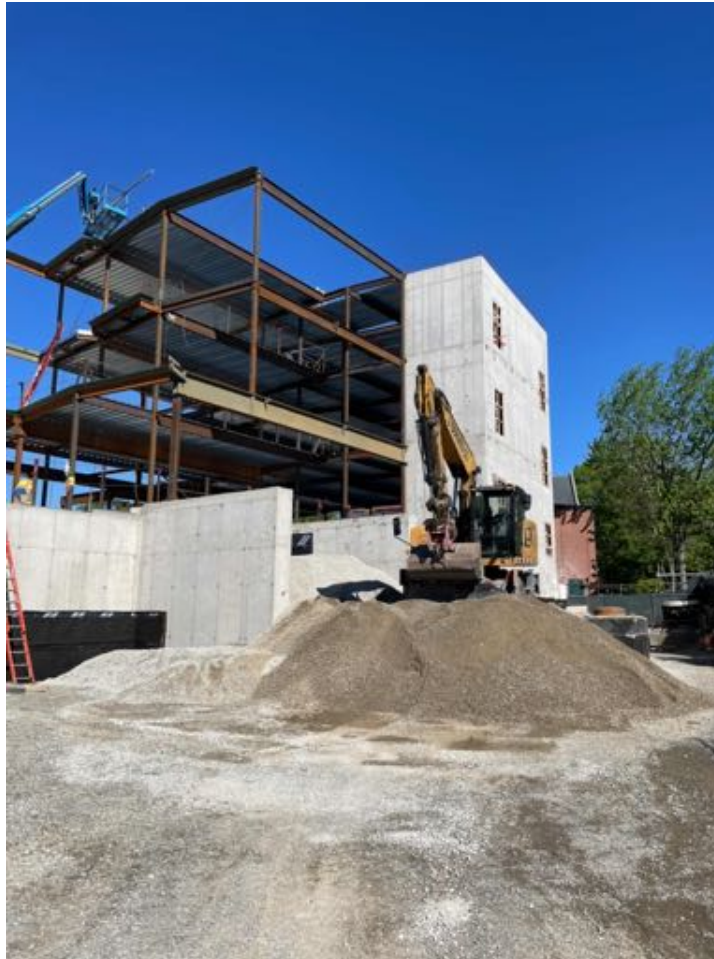
Backfilling, North side adjacent to Westbourne Terrace.
